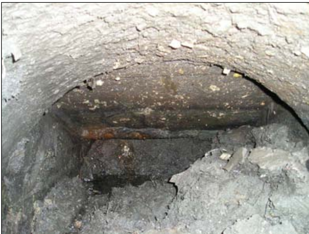
Figure 42. Sanitary Sewer from Bath House Built into Top of Clay Storm Drain, 1932.
