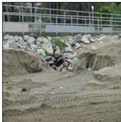
Figure 40. Overflow Stormwater Outfall at South Corner ICB
