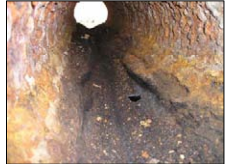
Figure 5. Leaking Sewer.
