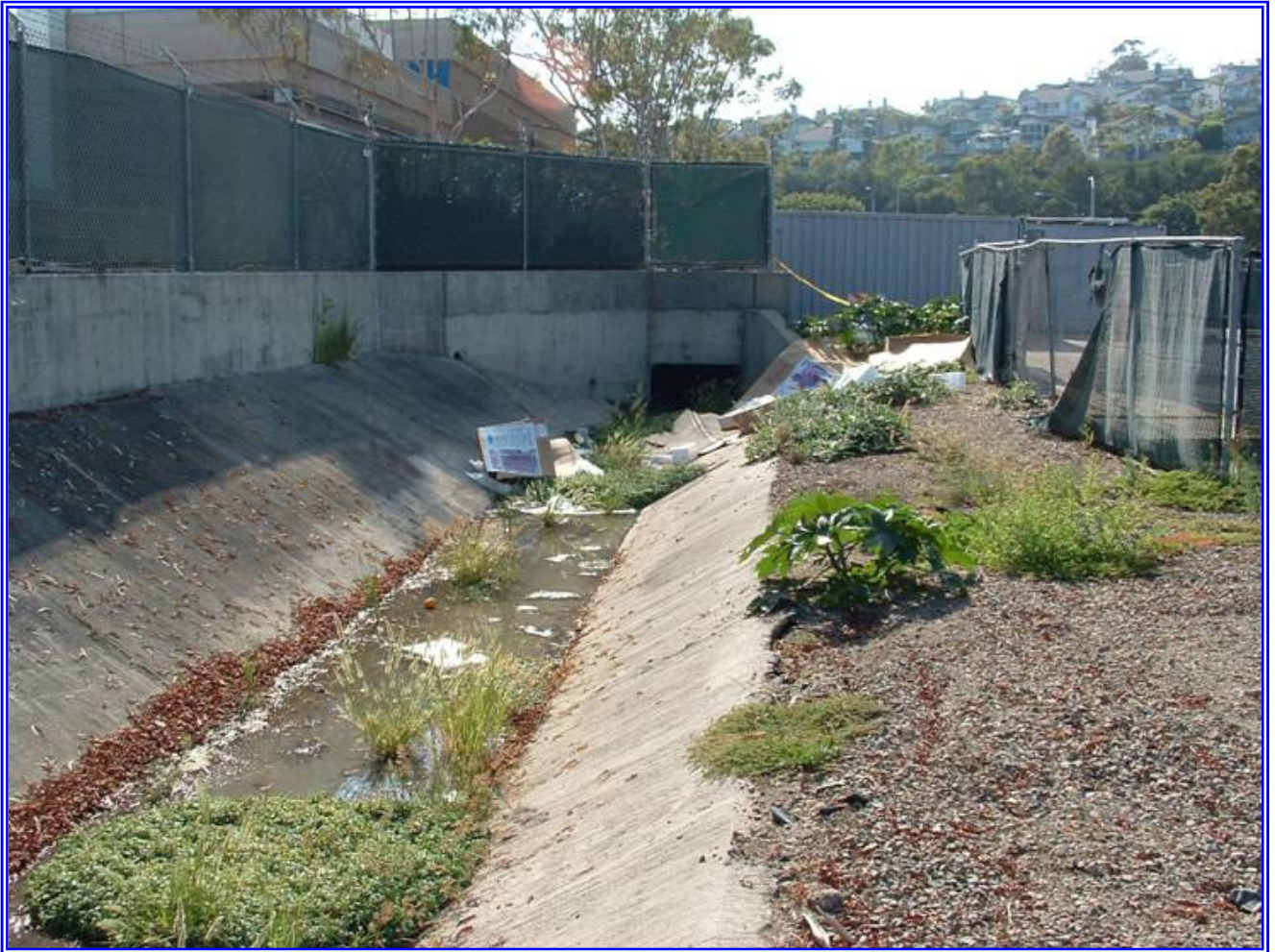
Figure 4.2 – Storm Drain Outlet Before Project Completion
