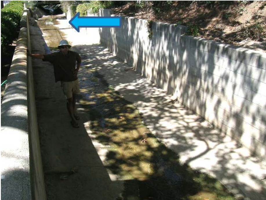
Figure 7. Site 1: Ramirez Canyon Creek Upstream of System
