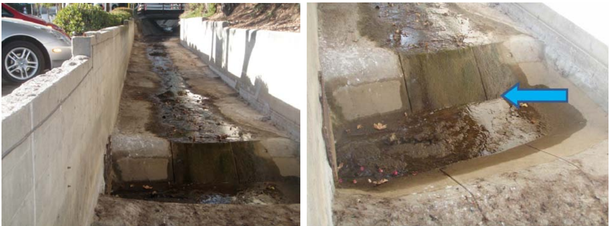
Figure 8. Site 2: Sump (prior to solids removal)
