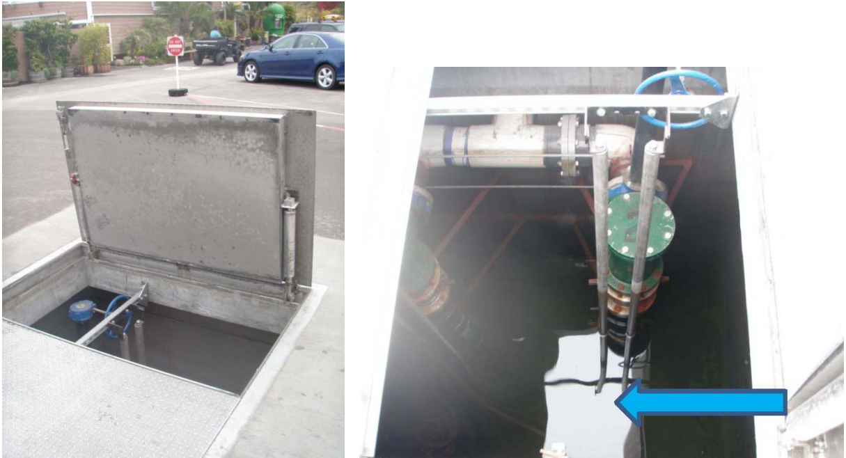
Figure 9. Site 3: Pump Station (post solids removal)
