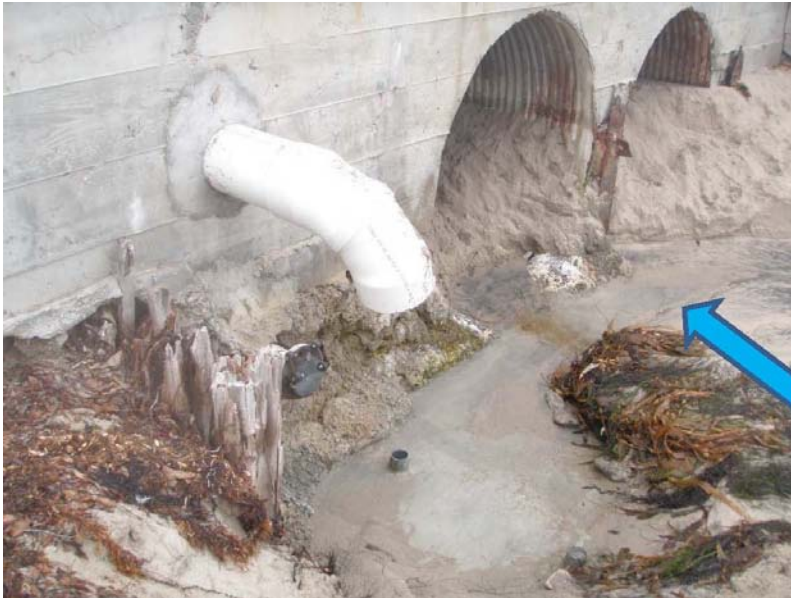
Figure 11. Site 5: At interface of treated discharge and the sand
