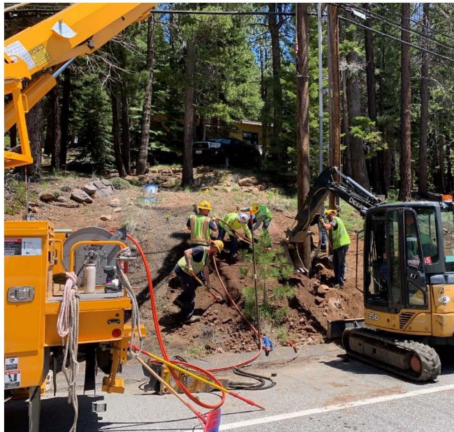
Figure 2: Truckee Donner PUD pole replacement in urban area that is a high fire threat area.
