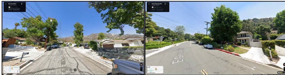
These Crescenta Highlands (left) and Glenoaks Canyon (right) locations are both within Tier 2 HFTDs. Utility activities managing the overhead power lines in these images would potentially be captured by the requirements of the Draft GO.
