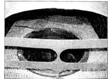
7. Place the chamber over the SedimenTrap™ and install the 10" PVC riser pipe as instructed on page 7.
