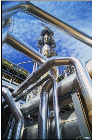
Wastewater Treatment Plant.
