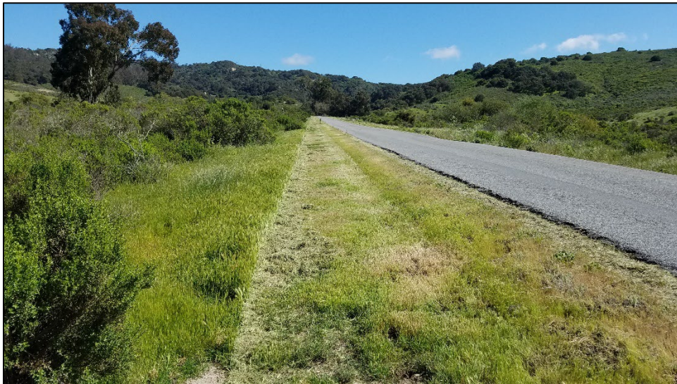
Photo A-8. View of Orcutt Hill Road and right-of-way in the southern segment of the proposed pipeline. Photo taken April 16, 2020.
