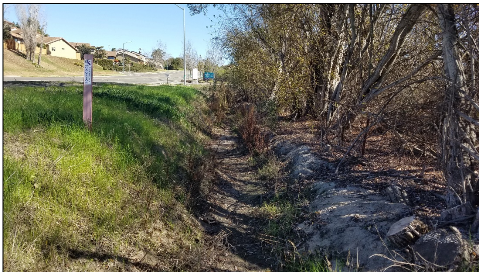
Photo A-8. View of Pine Canyon Creek reach that runs along East Rice Ranch Road. Photo taken February 10, 2020.
