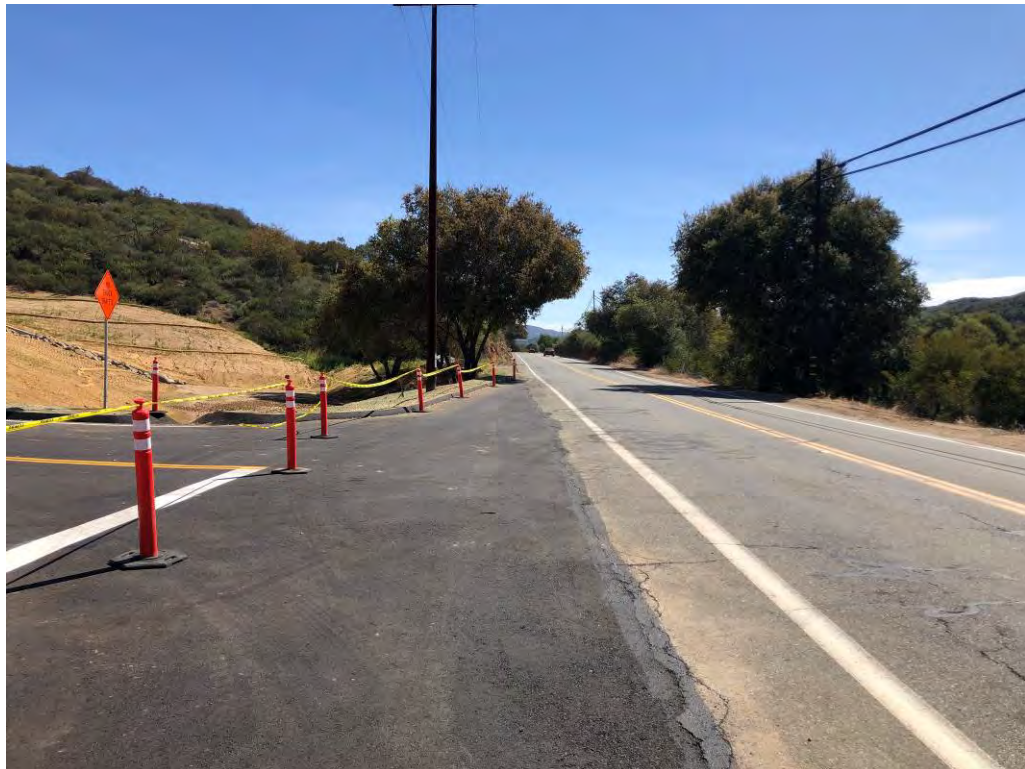
Photograph 4. View of APE near new Duro Road intersection, facing east.
