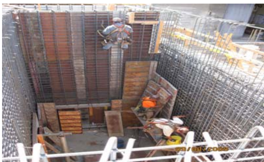
City of Palo Alto - Replacing UV disinfection facility
