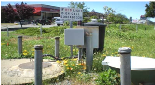
City of Colfax - Upgraded lift stations.
