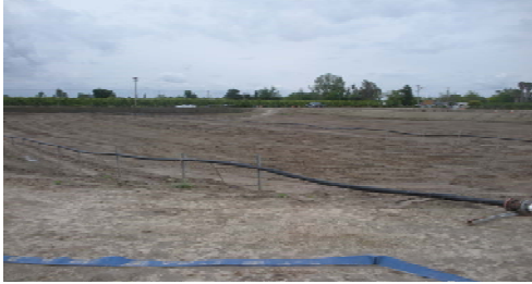
Construction of aeration pond
