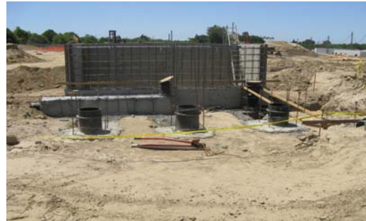
City of Hughson - Wastewater Treatment Site
