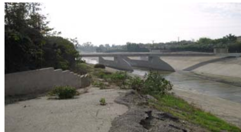
Pre-Construction View of Rain Garden location.
