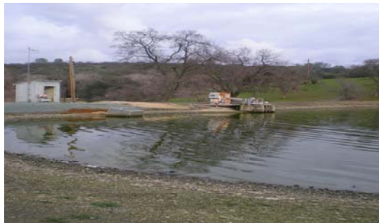
City of Plymouth - Improvement to the inflow/infiltration
