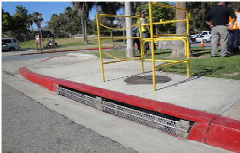
Installed Catch Basins
