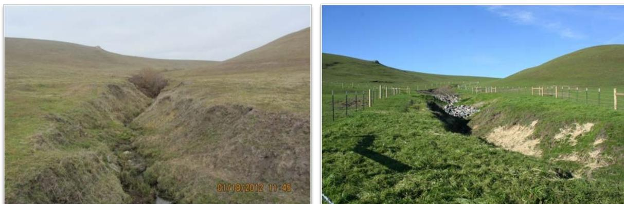
Figure 14: Pre-construction photo, left (1/2012) and post-construction photo, right (1/2015) – upstream view before and after riparian fence, grade stabilization, and revegetation
