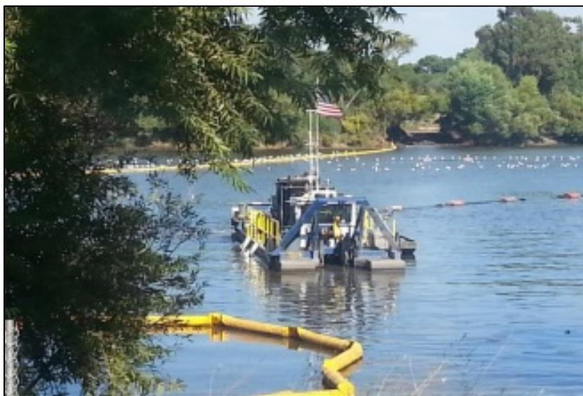
Figure 20: : Hydraulic dredging of contaminated sediments at Machado
