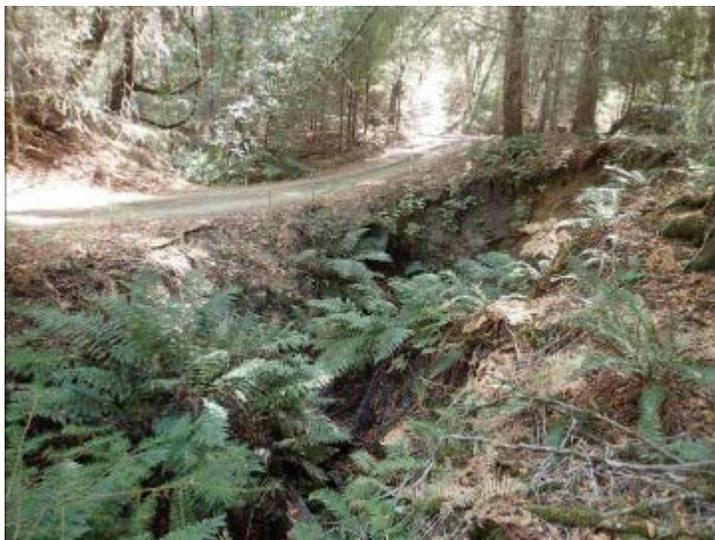
Figure 3: Pre-construction photo of a road crossing that blocks salmonid passage in the Navarro River Watershed. September 2, 2015
