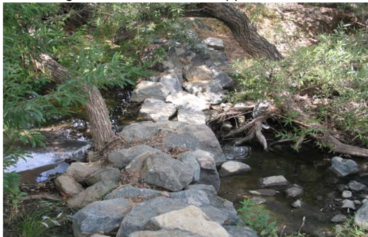
Grade stabilizer after installation and planting of riparian and wetland plants in spring of 2007.
