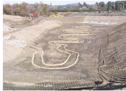
Fig. 3. First constructed wetland treatment cell after grading.
