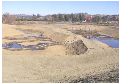
Fig. 5. Constructed wetland (1 st and 2 nd cells) during final grading.
