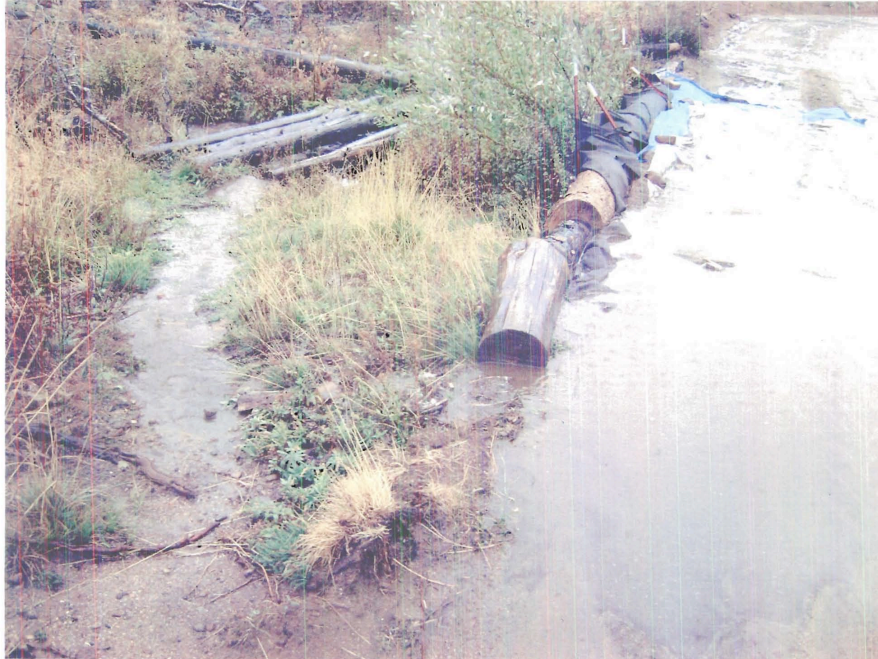
Photo 5: Sediment-laden stormwater discharging from road and crossing 11 into Angora Creek. No erosion control structures are installed.
