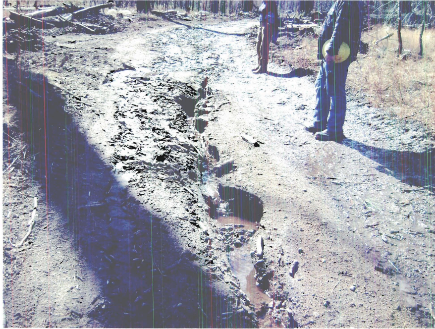
Photo 2: Forest Road 17E49, north of Seneca Pond in Unit 5 on October 15, 2009. No erosion control structures are installed.
