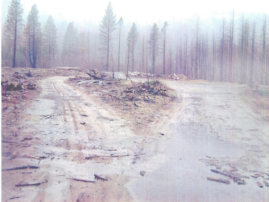
Photo 3: Landing near Seneca Pond in Unit 5 on October 13, 2009. Note lack of erosion control structures. Stormwater was running from landing, down road to discharge into Angora Creek (see Photo 4).
