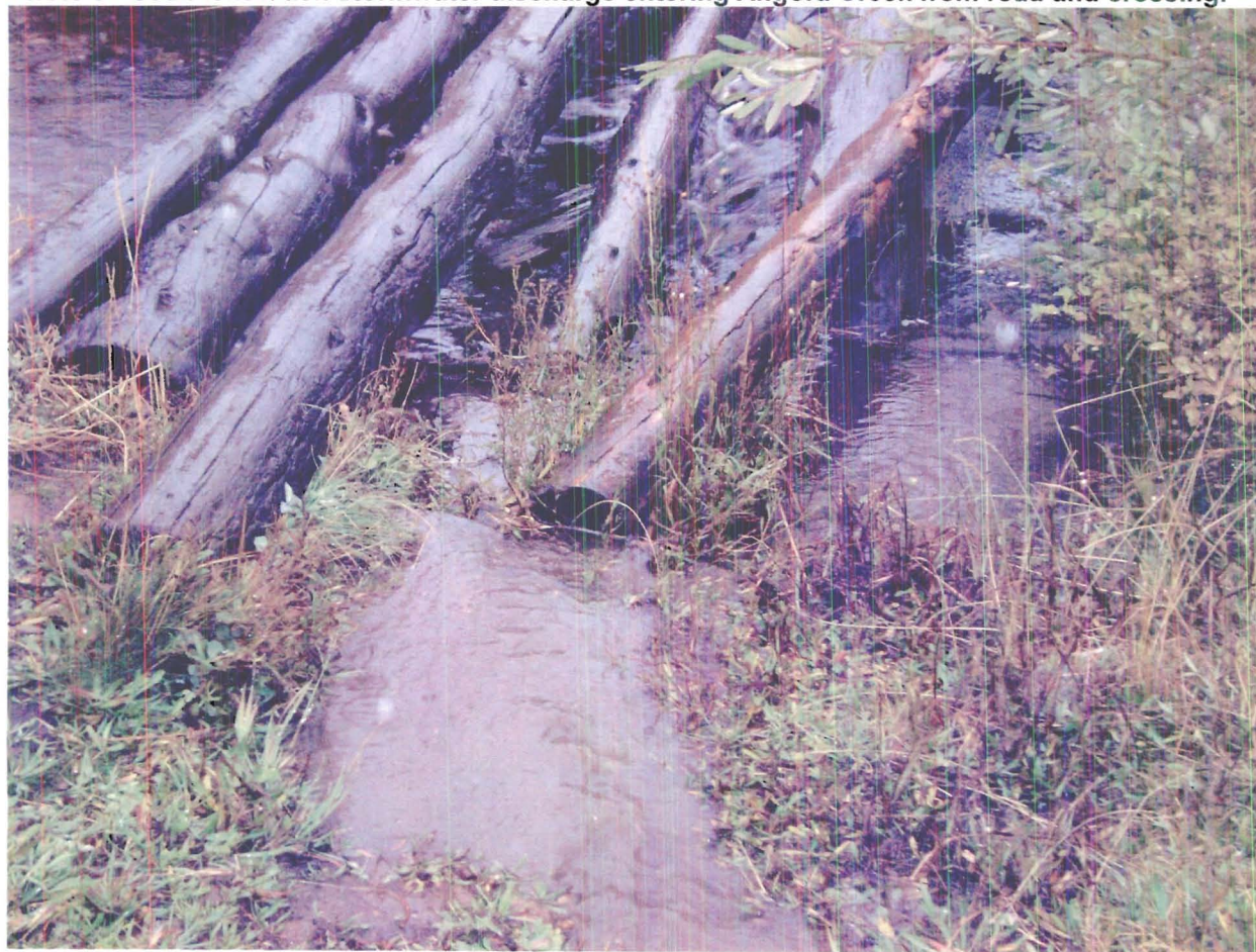
Photo 6: Sediment-laden stormwater discharge entering Angora Creek from road and crossing.
