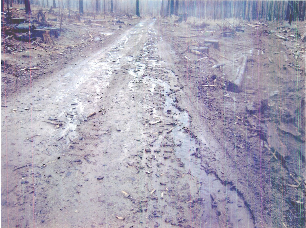
Photo 1: Forest Road 17E49, north of Seneca Pond in Unit 5 on October 13, 2009. No erosion control structures are installed.
