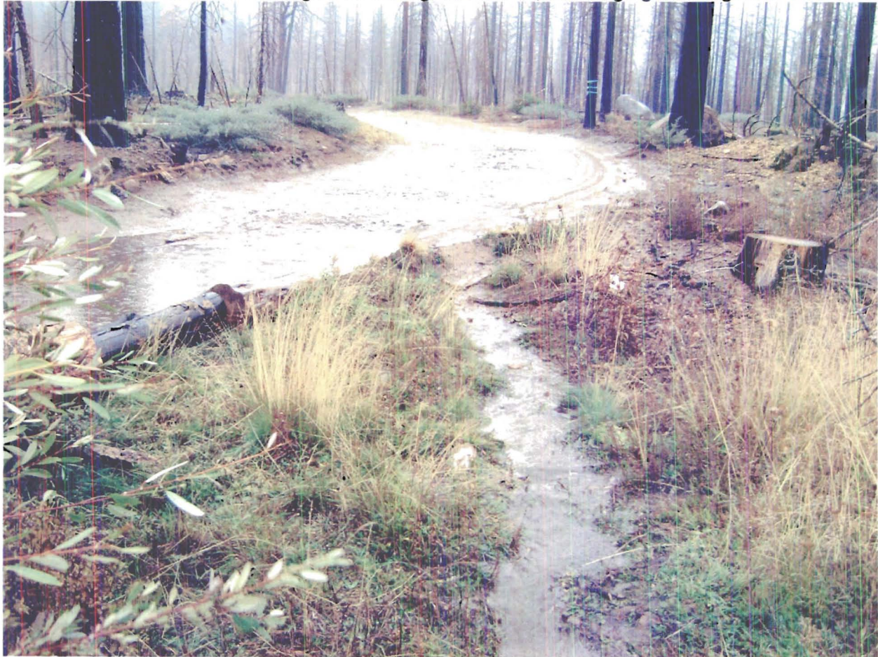
Photo 4: Road downslope of landing shown in Photo 3. No erosion control structures are installed. Stormwater was running from landing, down road, discharging into Angora Creek.
