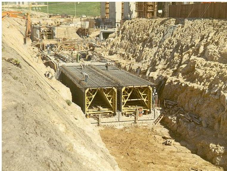
**Figure 11 – Original Circulating Water Tunnel Excavation & Construction**
