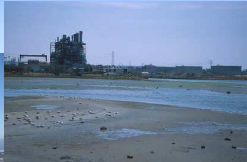
South Bay Power Plant (closed system)
