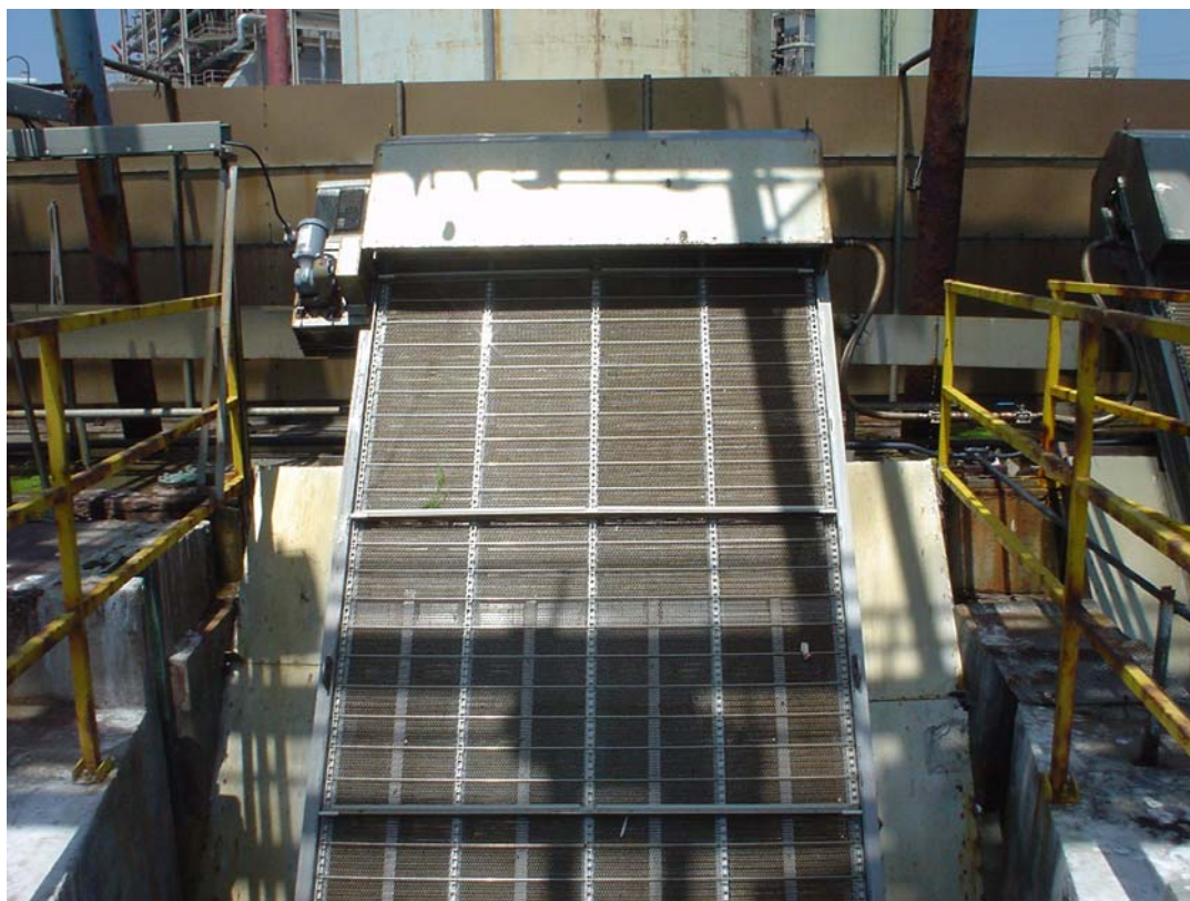
Figure 3.2-3. F.P.I. traveling water screens at the AGS.
