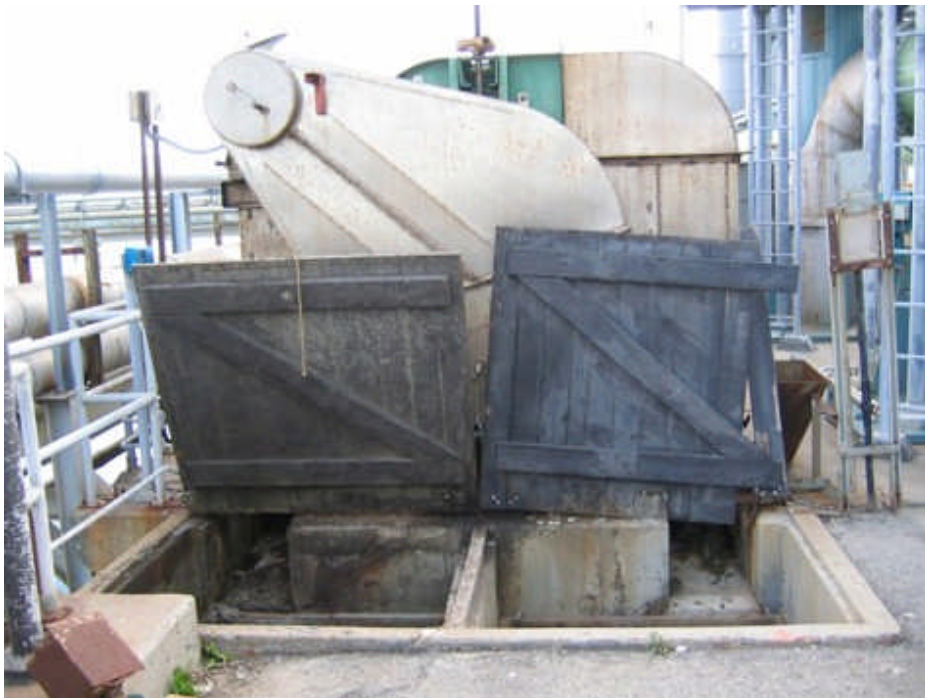
Figure B4-3. Units 3&4 (8-10) traveling screens sump collection area. The Unit 5&6 sumps are similar.
