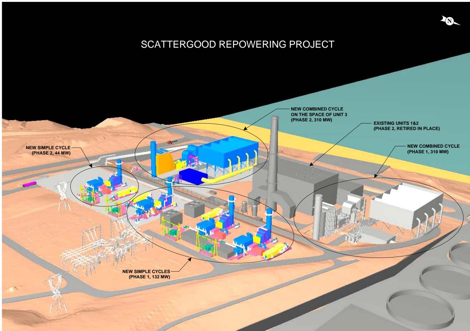
Figure SGS9 – Aerial View of Scattergood Generating Station Animated Final Layout
