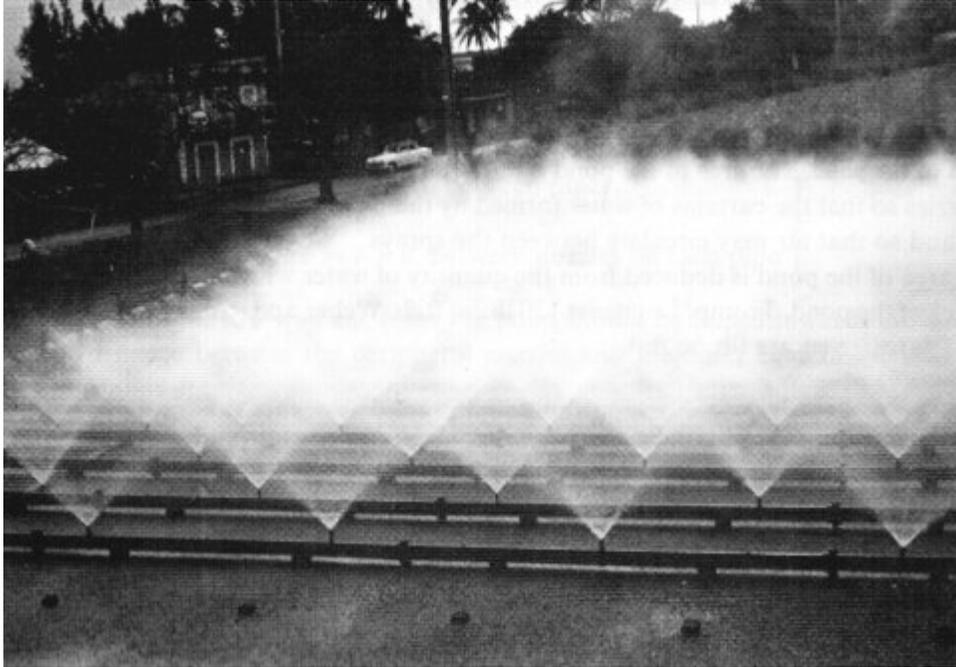
**Figure 6-28.** Visual example of a spray pond.
