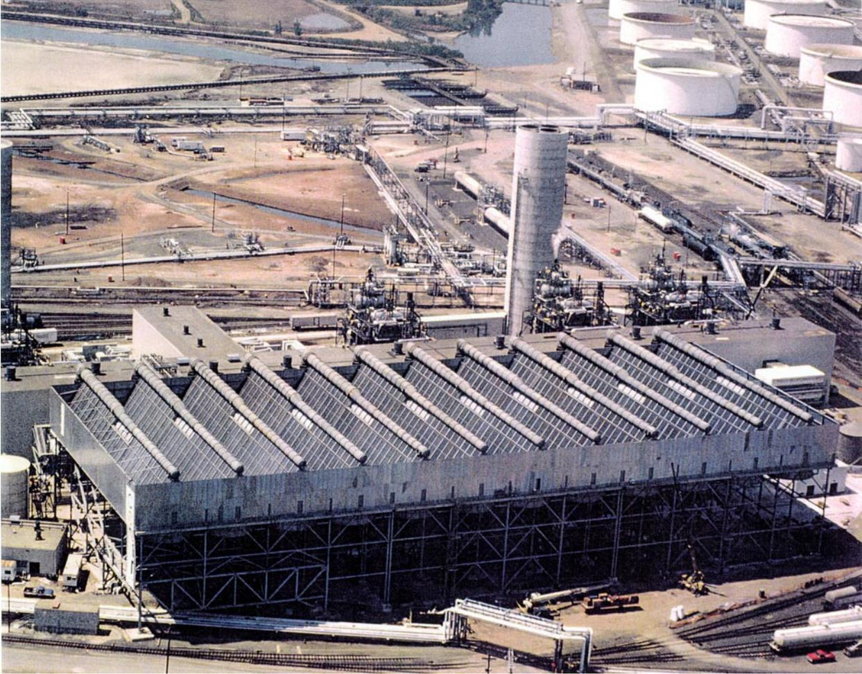
**Figure 6-31.** Visual example of an air-cooled condenser (courtesy of GEA).
