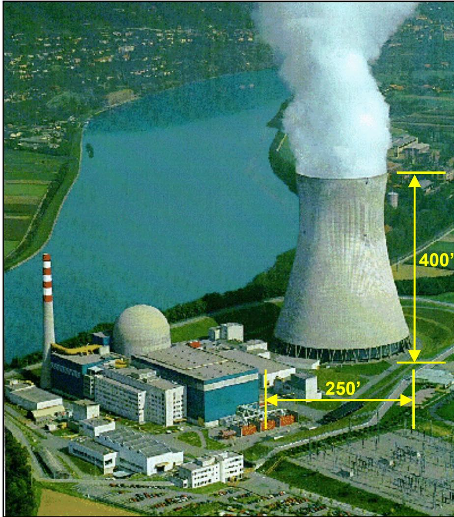
**Figure 6-24.** Visual example of a natural draft, hyperbolic cooling tower at a power plant facility.
