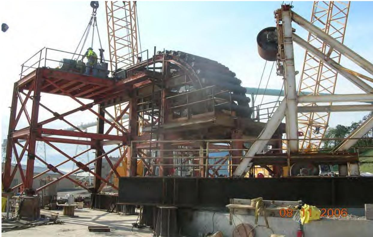
The TBM would begin boring operations, with the excavated material conveyed behind and vertically up the drop shaft to another horizontal conveyor belt, where it would be trucked away from the intake area:
