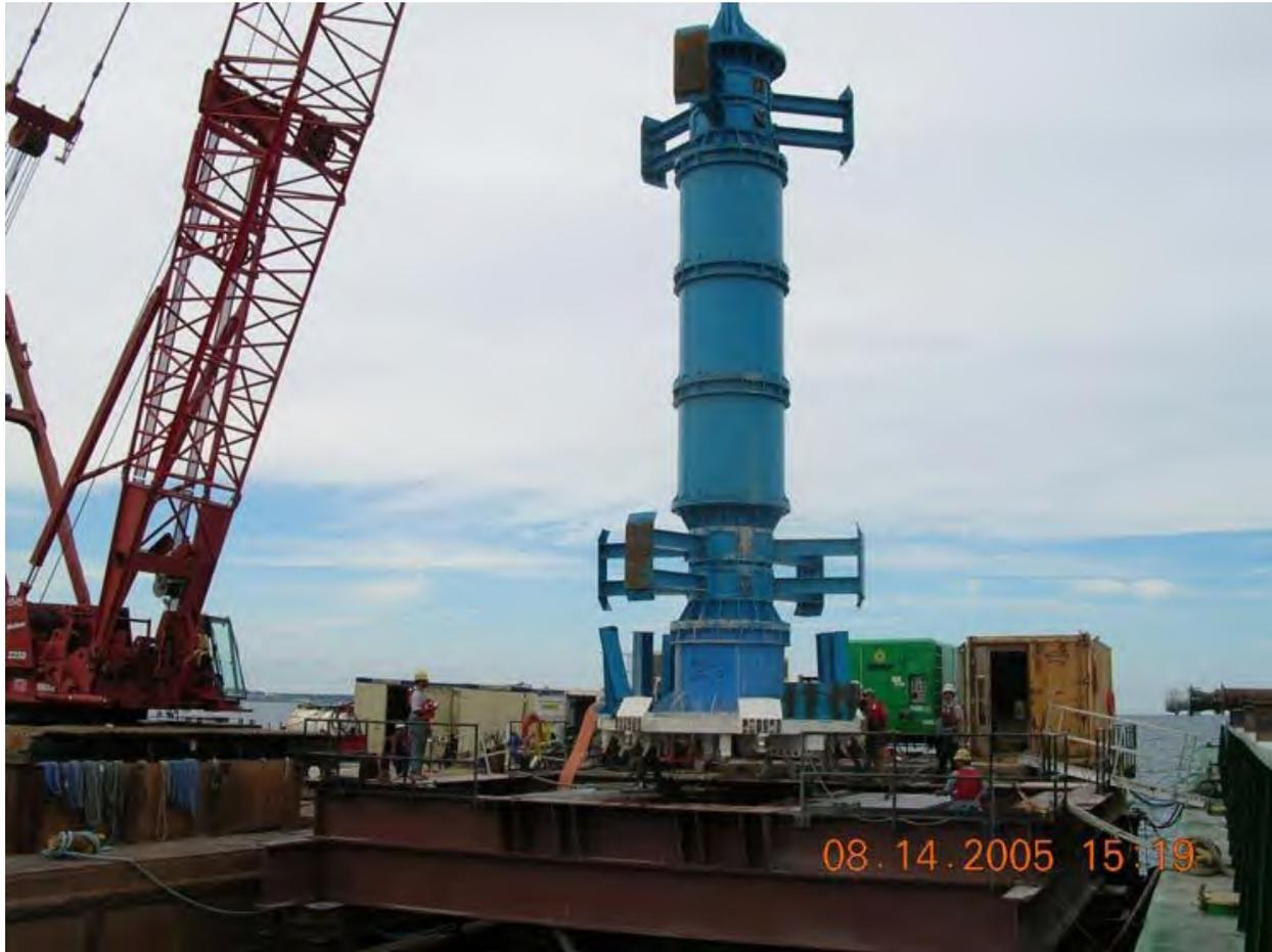
A 15-foot-diameter drill casing is then lowered inside the 18-foot conductor casing and reaches from the top of the sea bed down into the rock to form a seal.
