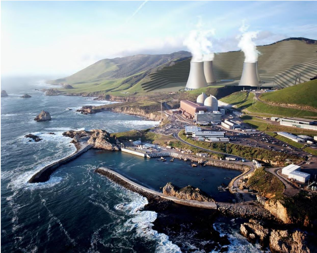
Figure 4.3-16. Wet Natural Draft Cooling Site Configuration
