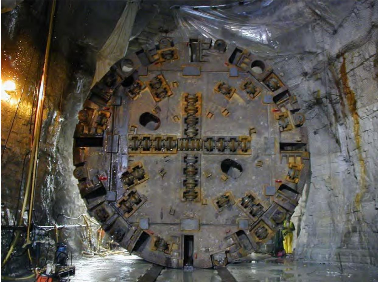
Once the TBM is assembled, the conveyor system would then be erected:
