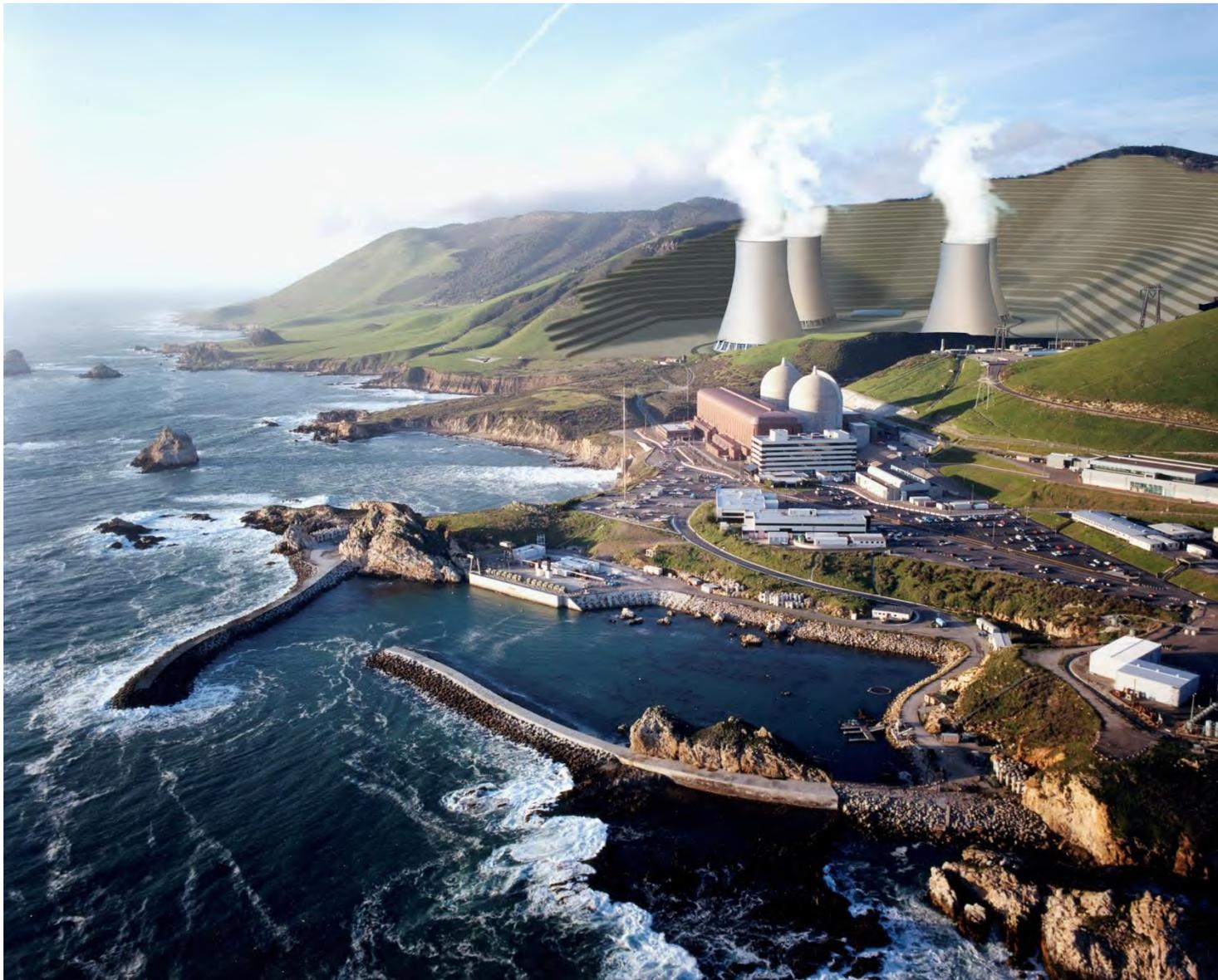
Figure 1-4. Plant Site Rendering Showing the Wet Natural Draft Configuration
