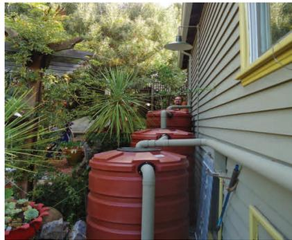
a good example. These are specially designed barrels placed underneath the downspouts of your house to capture rainwater from your roof. A hose can be attached so you can use it to water your yard! Another example of LID is a rain garden – a planted area of your yard where water either accumulates or slowly passes on its
