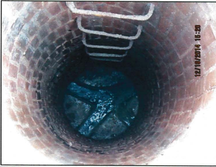
Photo 23: Manhole inspection (view 1); note heavy buildup on manhole base and in sewer line
