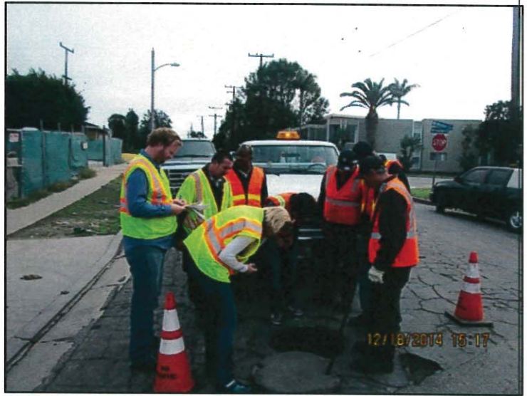
Photo 22: Manhole inspection (view 2)
