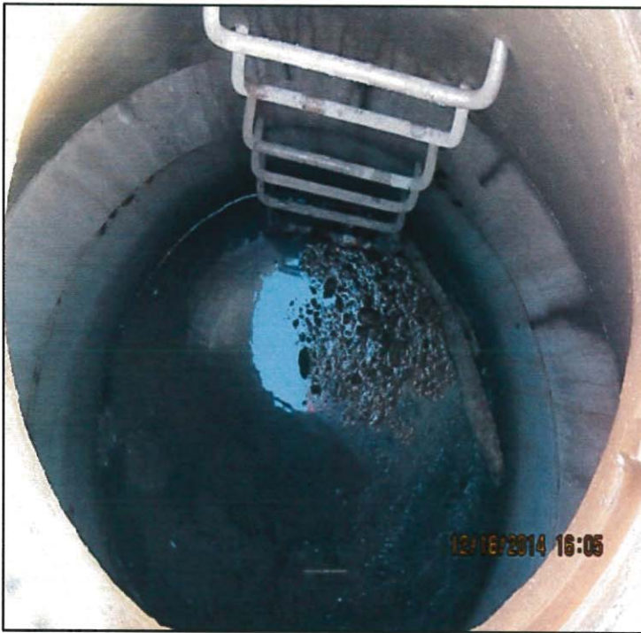
Photo 33: Siphon inspection (view 1); note heavy FOG mat on surface below
