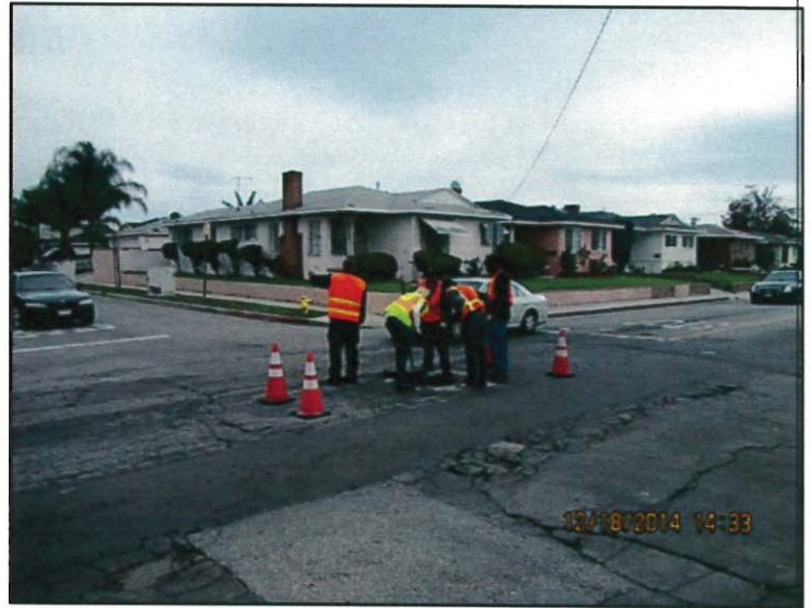
Photo 12: Inspection site (view 2)
