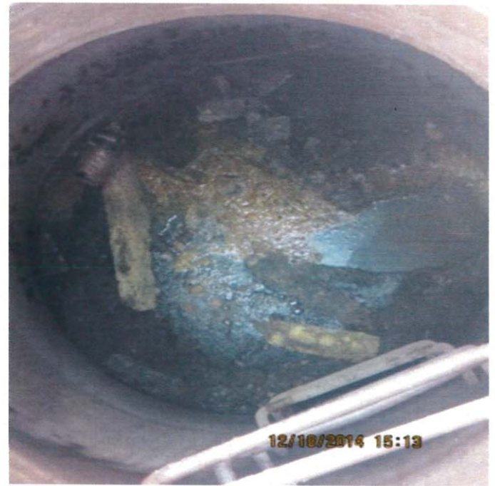
Photo 34: Siphon inspection (view 2); note heavy FOG mat on surface below
