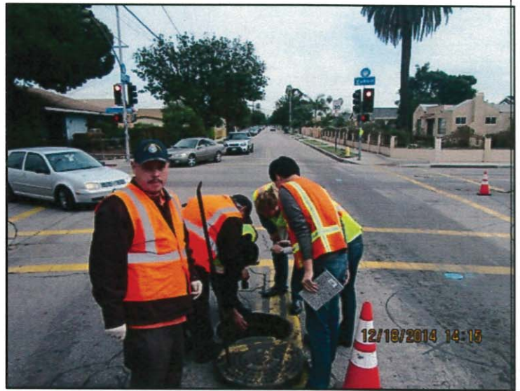
Photo 4: Inspection site (view 2)
