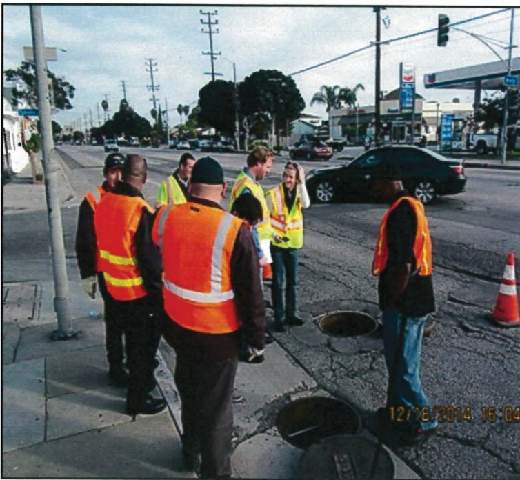
Photo 31: Sewer siphon inspection site (view 1)
