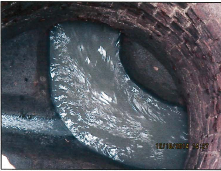
Photo 9: Manhole inspection; note LACSD trunk line on right with high flows
