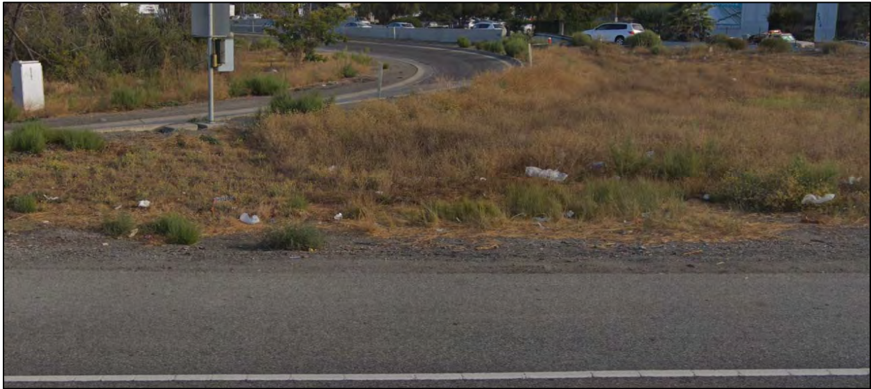
Figure 1: Partial Trash Capture by Vegetated Shoulder
