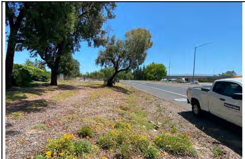
PHOTO B: Fill section with roadside vegetation strip slope flatter than 4:1 (sheet flow, 5'-10' to ditch) (SOUTH)
