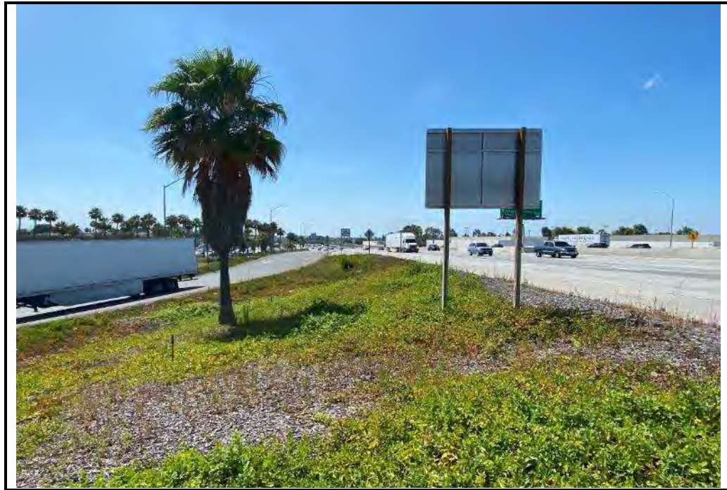
PHOTO C: Fill section with roadside vegetation strip slope between 2:1 and 4:1 (diked/curbed, 5-10' to ditch) (SOUTHEAST)
