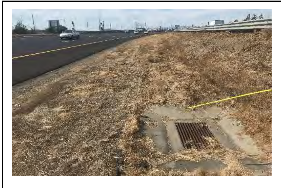
PHOTO A: CAPTURE DEVICE LOCATION (DROP INLET)
