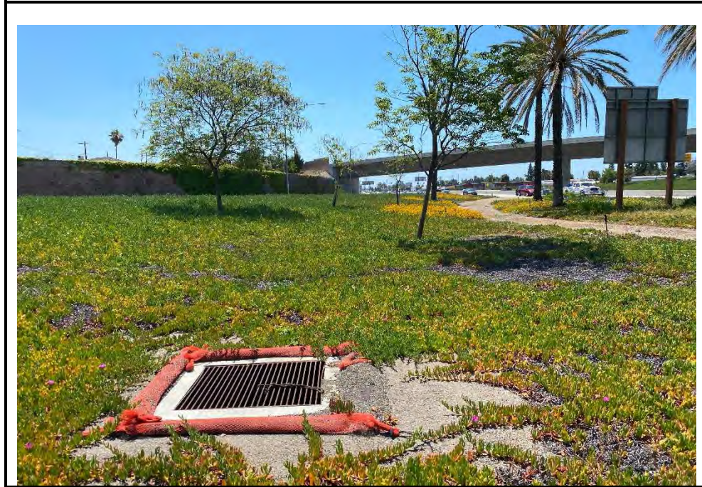
PHOTO A: Fill section with roadside vegetation strip slope flatter than 4:1 (diked/curbed, 10'-20" to ditch) (SOUTHWEST)
