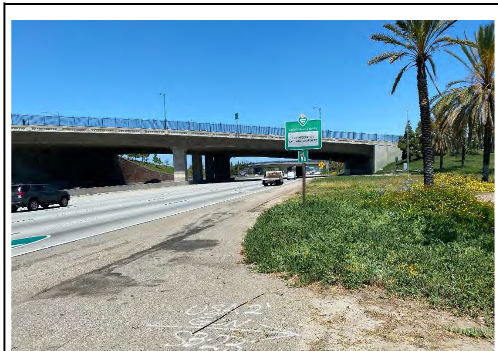
PHOTO B: Fill section with roadside vegetation strip slope flatter than 4:1 (diked/curbed, 10'-20" to ditch) (NORTHEAST)
