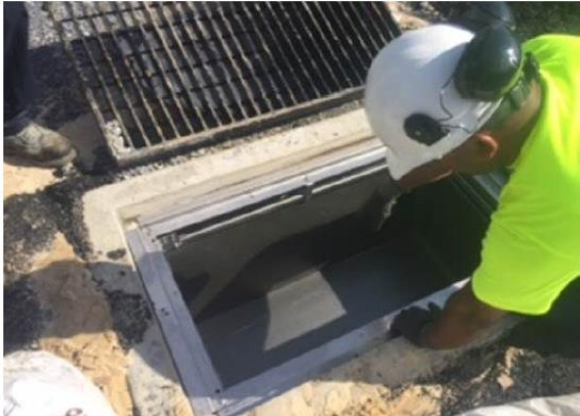
Photos 3,4: FTC inserts shown during installation into a catch basin
