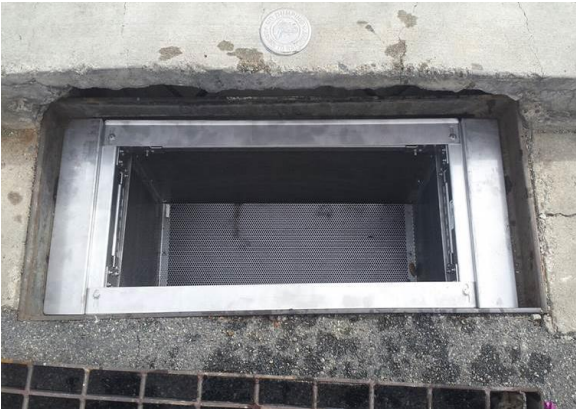
Photos 3,4: FTC inserts shown during installation into a catch basin
