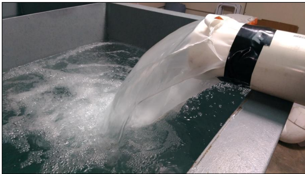
Figure 4. Net at effluent pipe discharge.
