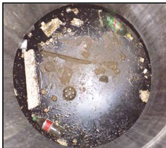
Floatable debris in the Aqua-Swirl ®
