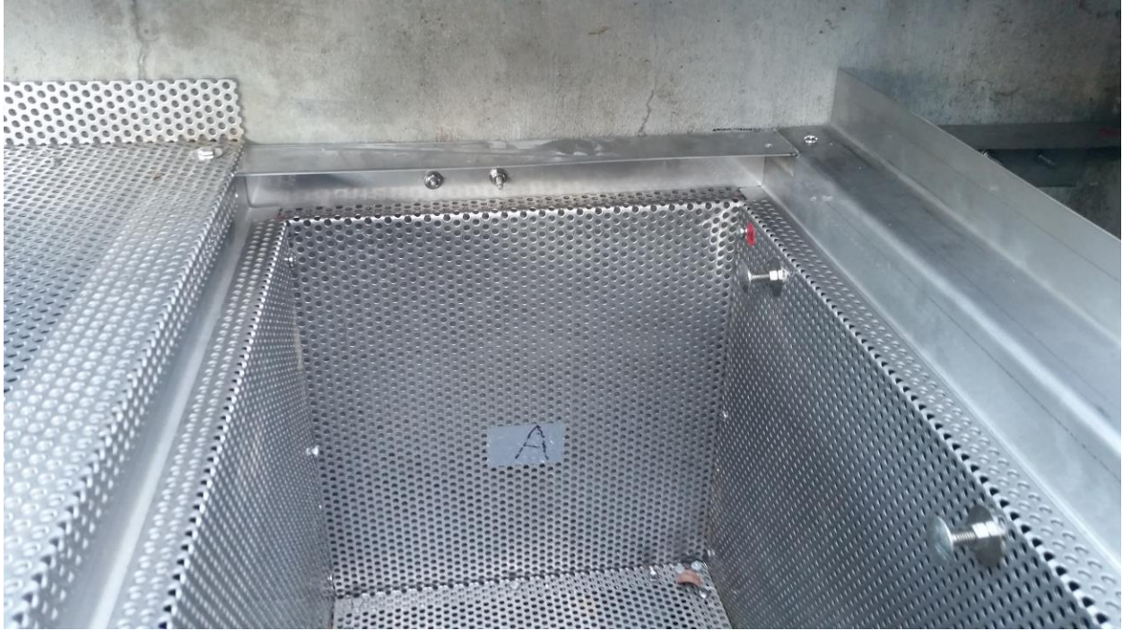
Figure 4. Installed Curb Inlet insert 100% connection at rear vault wall
