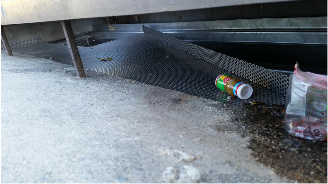
Figure 2. Installation of Curb Inlet insert and vector control access point behind perforated pan
