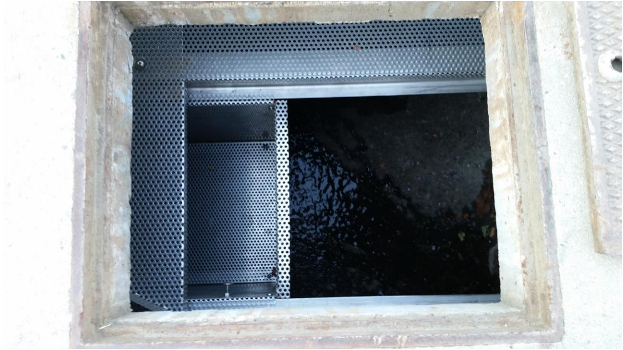
Figure 6. Collection basket view through manhole during vault cleaning and maintenance; vector control access point ; jetting, cleaning, camera and confined space services accessible without removing parts
