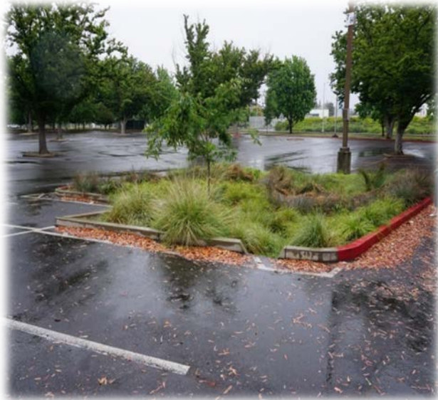
Figure A: CA State University-Sacramento Bioretention BMP
