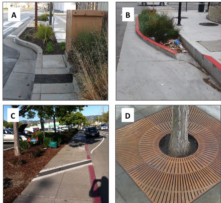
Figure 1. LID designs with high (A), low (B) and intermediate (C) angles of storm water entry; and LID with a screen design feature (D). Image credit A. Gilbreath (A-C) and Iron Age Designs (D).
