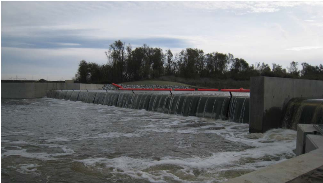
Figure 2-3: Rubber Dam with Gate Installation, Salinas, CA
