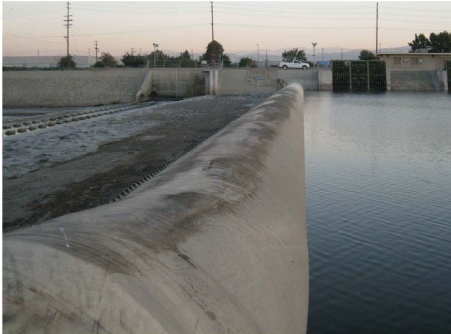
Figure 2-1: Traditional Rubber Dam Installation, Imperial, CA
