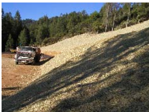
straw cover erosion control
