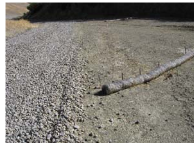
rocked road and wattle to reduce erosion at City Landfill
