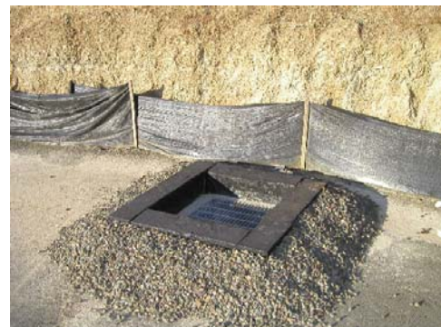
protection of drop inlet with rock & silt fence
