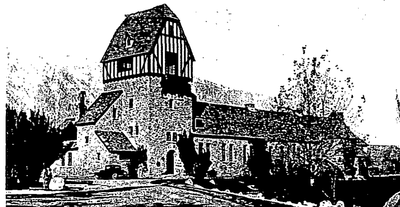
FIGURE 34. Mount Whitney Hatchery, completed in 1917. Built of massive chunks of native stone, with the towering Sierra Nevada in the background, it is a symbol of ruggedness.
