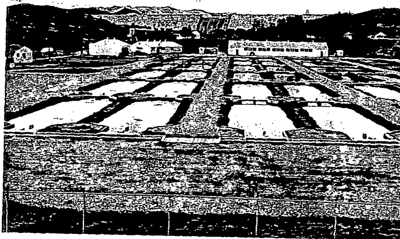
FIGURE 45. Standard California type earthfill rearing ponds, San Joaquin Hatchery. The ponds are 100 feet long and are arranged in series of 6 ponds. Each series requires 3½ cfs of water. Friant Dam, which forms Millerton Lake, is in background. Photograph by William M. Carah, May 1956.
