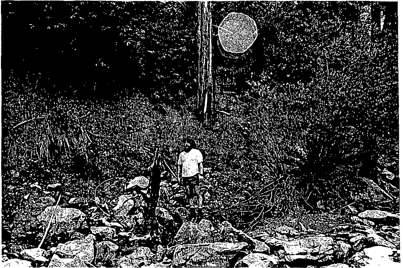
Figure 4. August 1983 photograph showing an example of aggradation from 1964 flood which buried and killed trees on former streambank.
