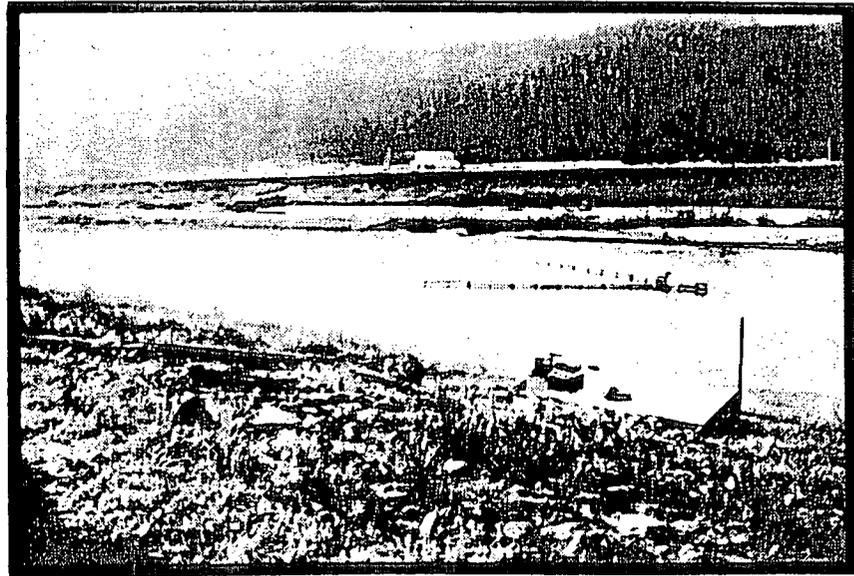
Figure 4. Rear Section of Weir Showing Adjustable Panels with Inclined Plane and Removable Holding Bucket (upper), and Weir in Redwood Creek, 1983 (lower).
