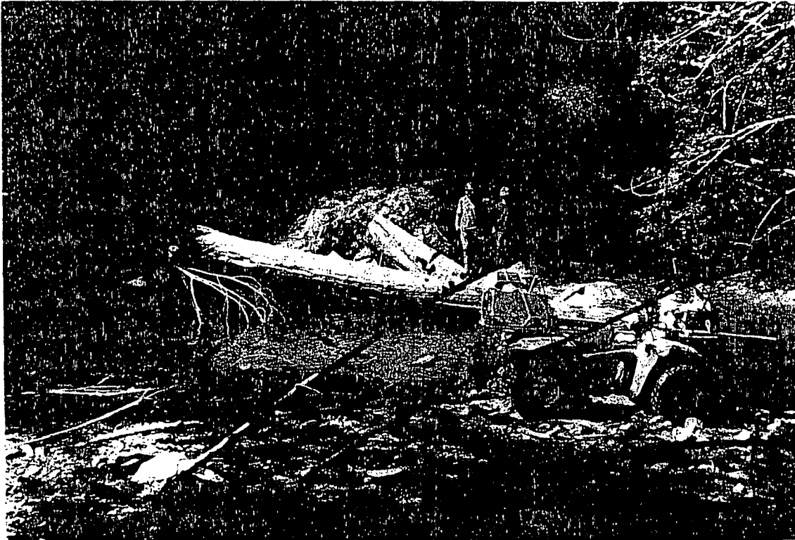
1996 completed LWD Cover Structure
