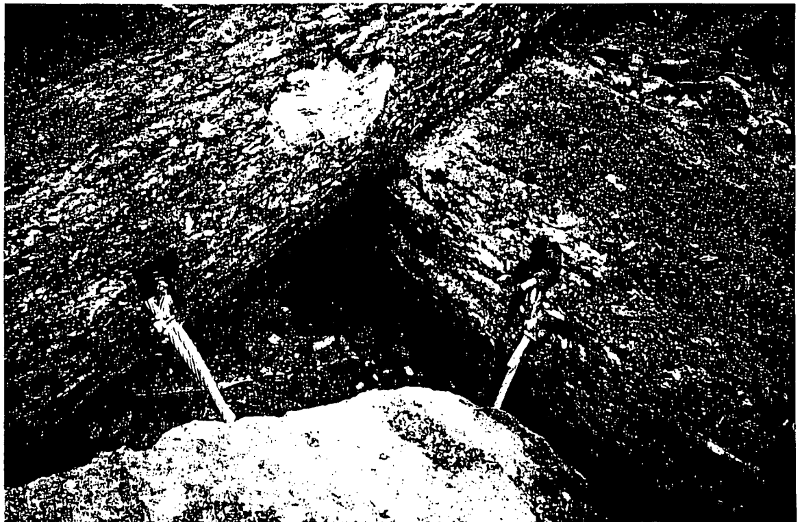
Cable eye to threaded rebar anchors securing LWD to boulder
