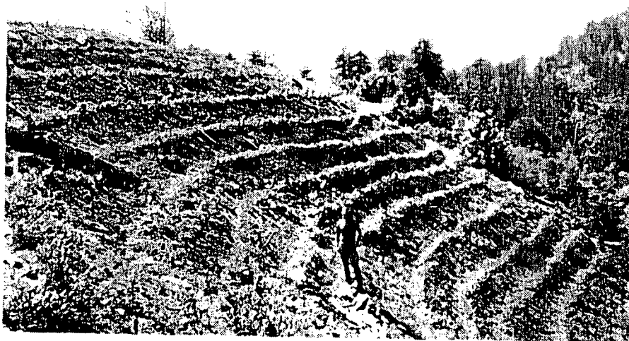
Fig. 2. Slope protected by contour wattling. Partially buried and staked willow wattles protect slope against erosion. Wattles root and sprout thus further stabilizing slope. Redwood National Park, California.
