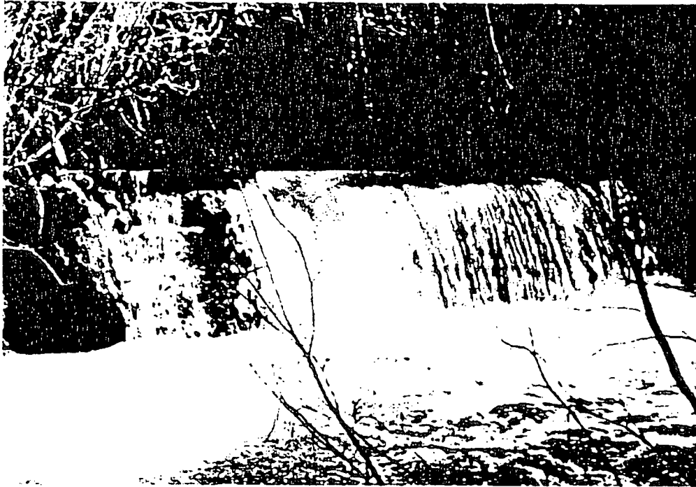
FIGURE 10. Abandoned dam on Olds Creek, 1/4 mile upstream from mouth prior to correction. This was a partial barrier to upstream migration of fishes. Photo by Gerald Holman, January 6, 1960.
