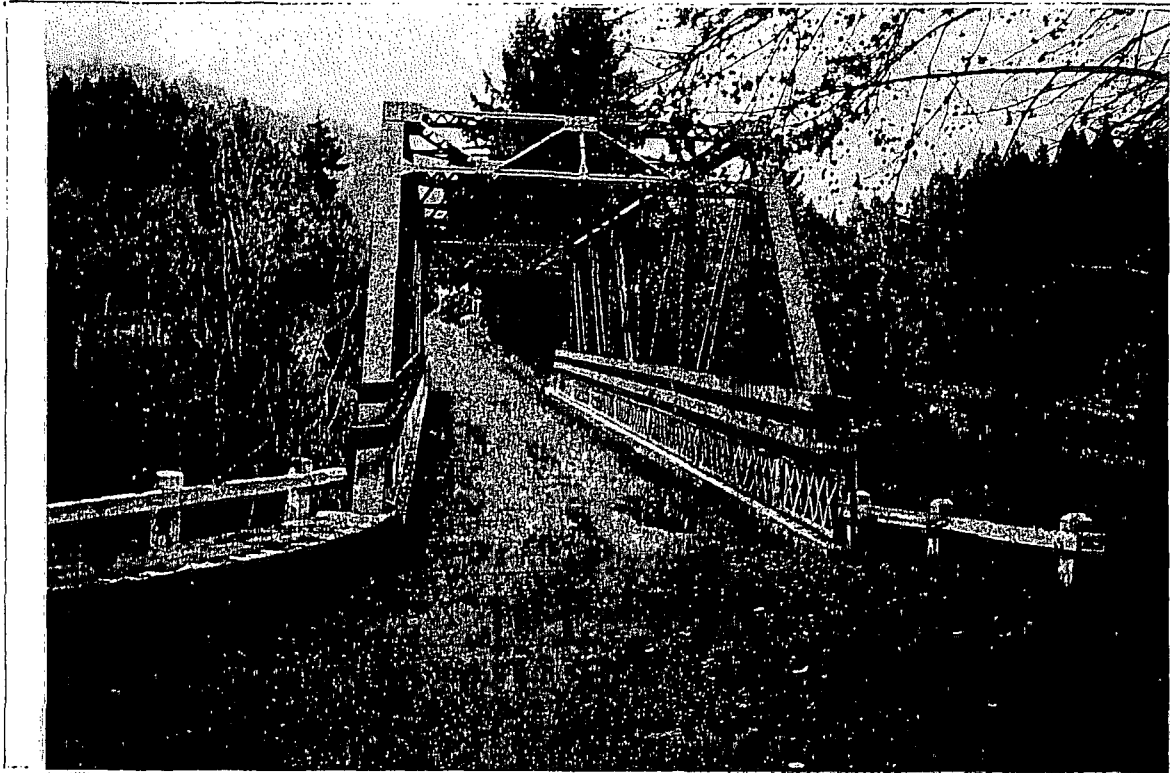
Approach Roadway Looking * West
