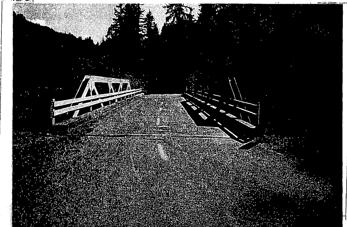
Approach Roadway Looking * South
