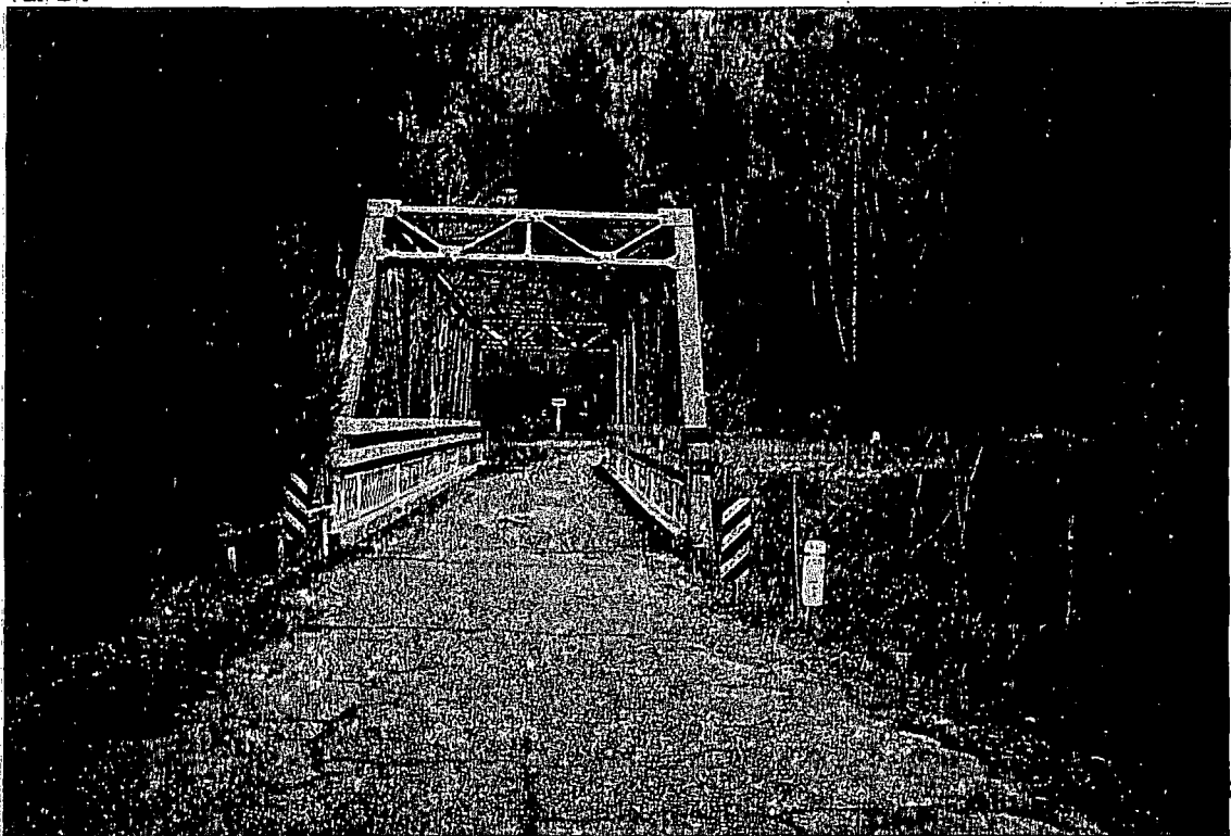
Approach Roadway Looking * East
