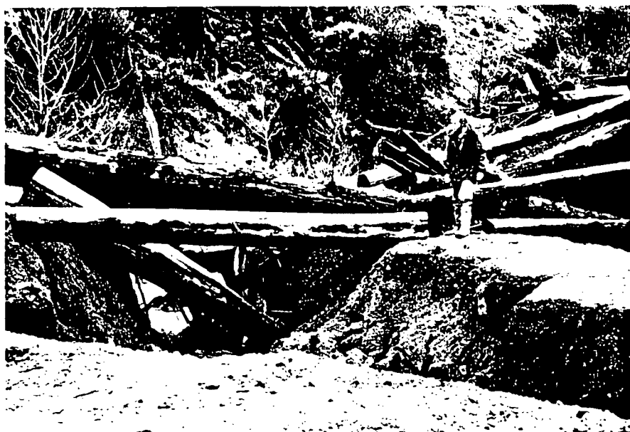
Photo 20. An earth and log bridge which washed out during the winter of 1968-69 was not repaired or removed even though the road beyond was impassable. An estimated 100 cubic yards of earth once filled these cavities. Location is at mouth of Last Fork 1 (April 1971).
