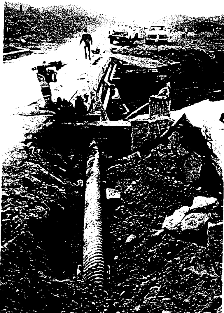
View, looking south, of sewer main repairs in progress. Section of corrugated metal pipe in foreground that encased force main where it crossed bridge.
