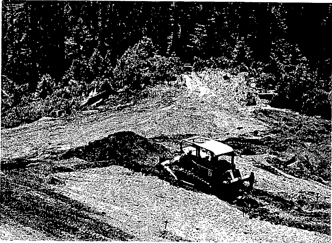
Figure 1. Bulldozer mixing compost into ground.
