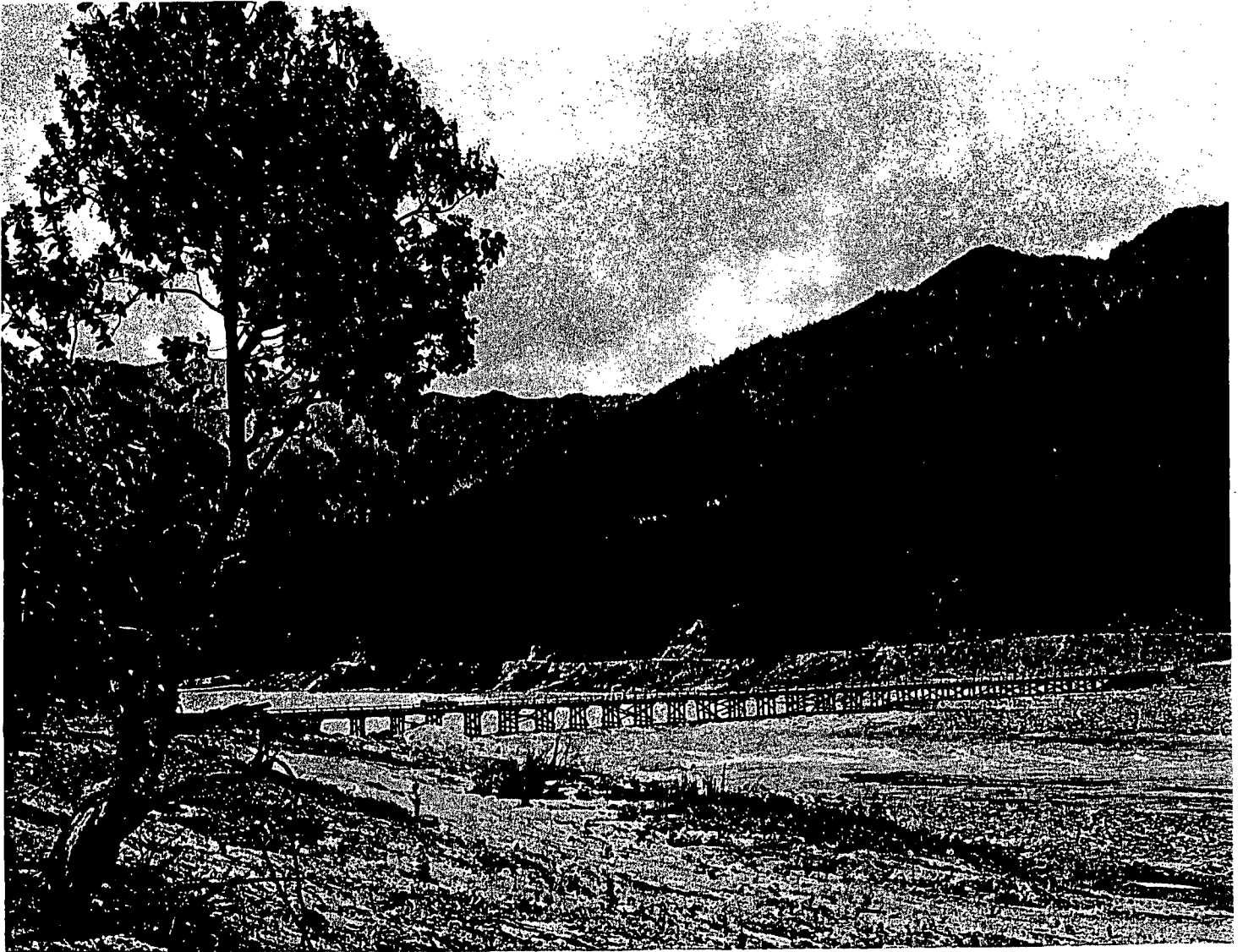
Temporary low-level bridge at Orleans to carry traffic while new bridge over Klamath is being constructed. This will be a major project.
