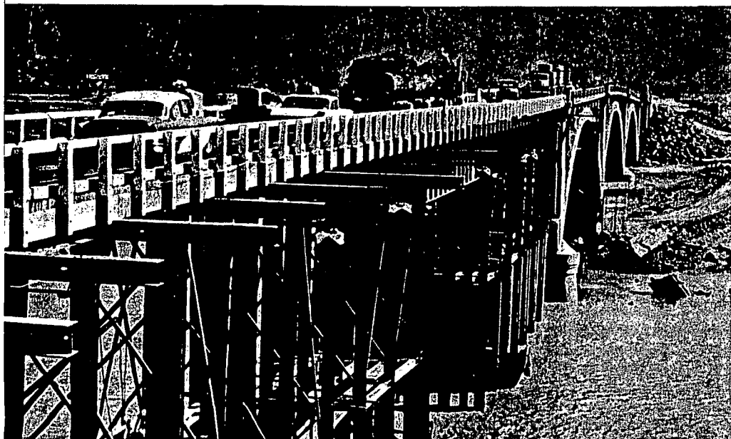
Klamath River Bridge with temporary repairs, opened to traffic on March 14, 1965.
