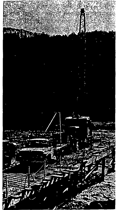
ABOVE: First stages in construction of temporary crossing over Klamath River to replace washed-out Orleans suspension bridge. BELOW: Construction stage on replacement bridge at Somesbar. With abutments and pier intact, girders were quickly positioned to replace truss which stream carried away.
