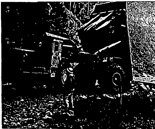
Fortunately, several contractors already had big rock trucks such as this in the vicinity, and they were invaluable in replacing road base.
