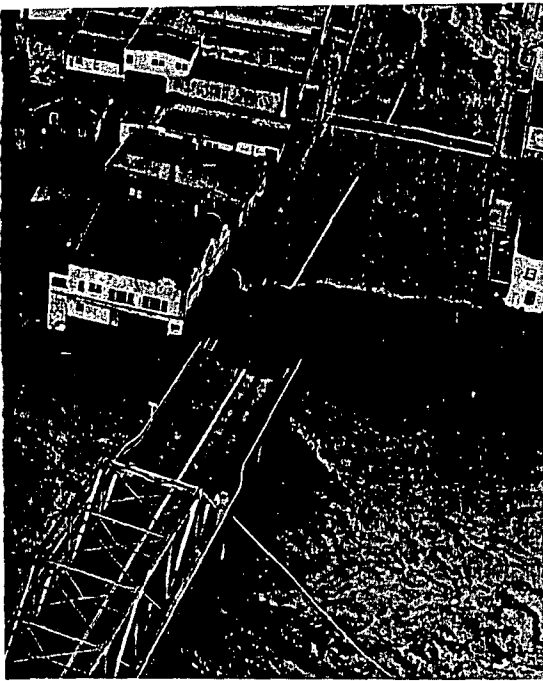
ABOVE: North abutment of North Scotia Bridge at Rio Dell torn out by force of Eel, here shown partly in flood. Building at left of broken bridge end is now gone. (Photo courtesy of Eureka Newspapers, Inc.) BELOW: Looking south along US 101, the Redwood Highway, with the town of Klamath in the foreground, and washed-out bridge in the background. (Photo courtesy of Eureka Newspapers, Inc.)
