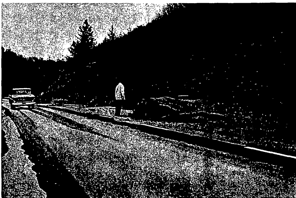
ABOVE: This paving damage was caused by pressure of sliding material on slope at right, forcing its way between road surface and foundation. BELOW: Man in photo has right hand at high-water mark which South Fork of Eel reached here near Phillipsville. This stretch of freeway, recently completed, was constructed five feet above high-water line of 1955 flood.
