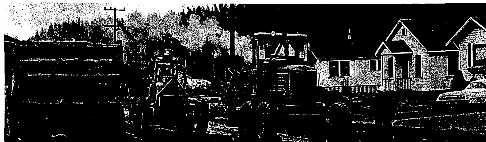
ABOVE: Amount of fill required to repair such slipouts was dependent upon how far down "toe" of slope lay. BELOW: Grader, front-end loader, and dump trucks work together to remove silt in Orick, several feet deep in places, as can be seen beyond highway shoulder.
