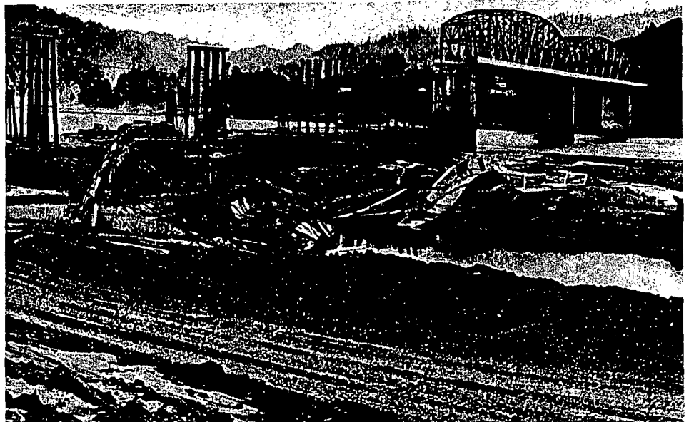
Repairs going forward on Robinson Ferry Bridge over the Eel. Crews gambled stream would not flood again this winter, and as payoff bridge will be opened to traffic in May. Wreckage of old spans lies in center foreground.
