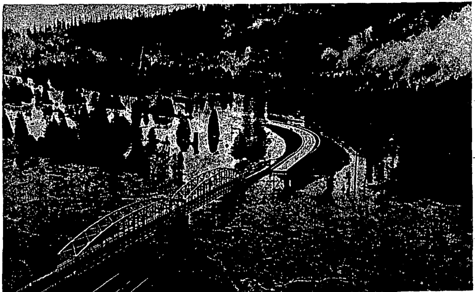
ABOVE: Debris deposited by flood on US 101 in redwood groves just upstream from Pepperwood. Barn with cupolas came from site across river and several miles upstream. BELOW: Downstream bridge of pair on Redwood Highway at South Scotia was also flood victim. Older bridge at left of through-truss design, survived flood because it was high enough to avoid debris which collected on truss below deck of newer bridge now missing at right. (Photo courtesy of Eureka Newspapers, Inc.)
