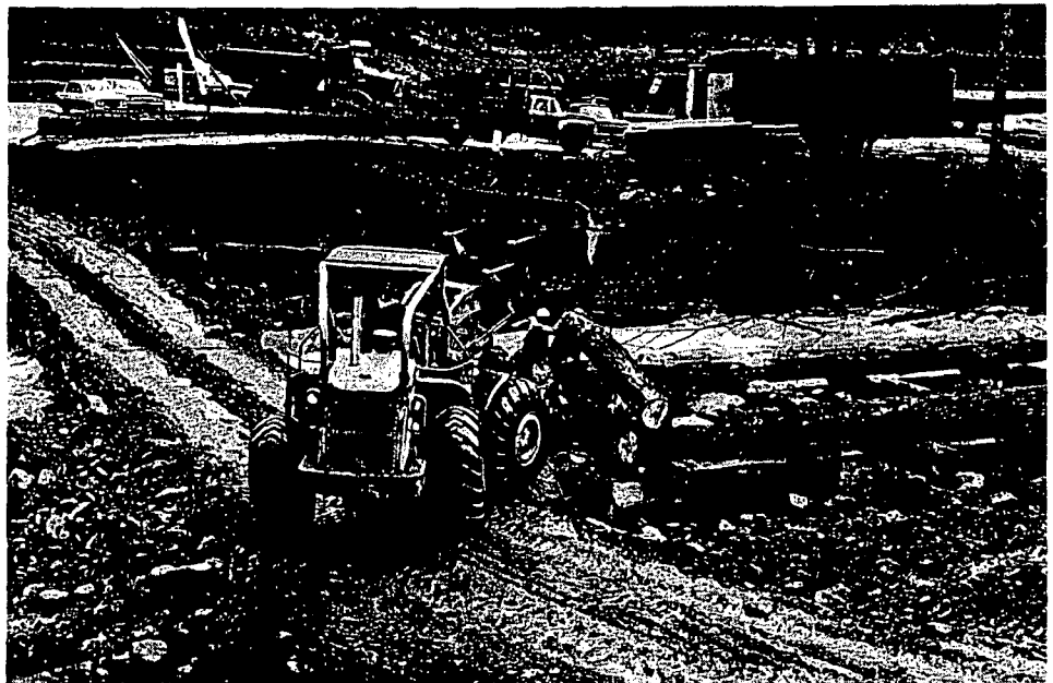
ABOVE: After first building low-level log bridge to move equipment in, contractor here, using front-end loader as crane, puts logs in place for abutment for higher level crossing. BELOW: The finished bridge, crossing Patrick's Creek, US 199.
