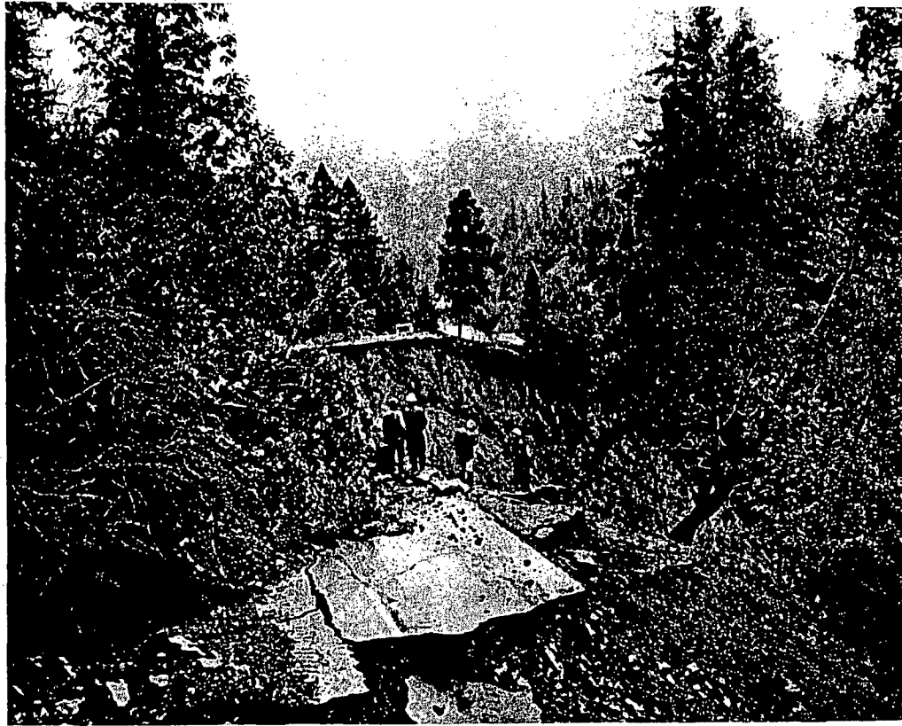
Gaping washout from what is normally an insignificant trickle of a stream is typical of damage throughout the several northwestern counties in the December 1964 floods. This is State Route 208 in Mendocino County, west of Leggett.
