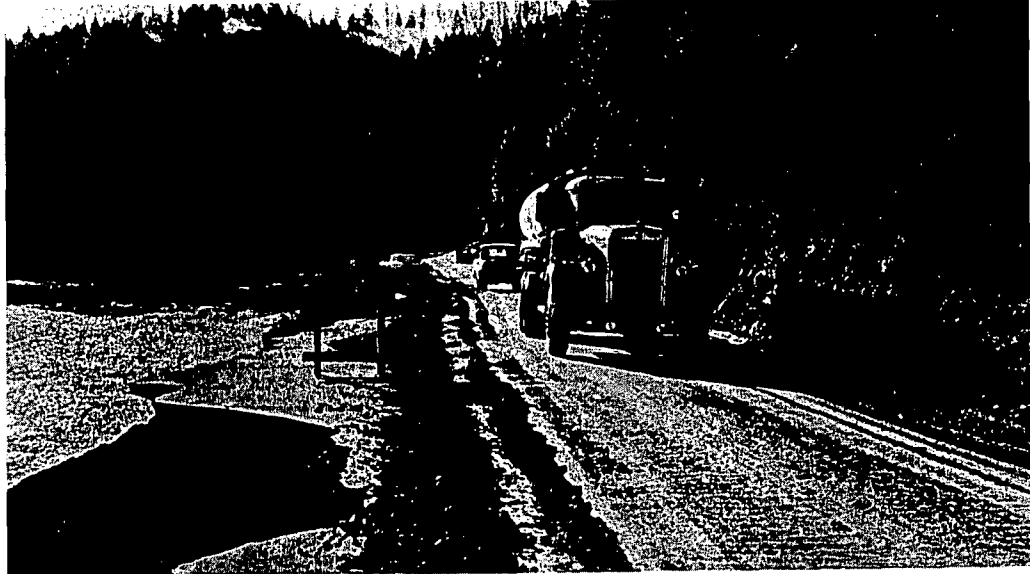
Section of Redwood Highway south of Pepperwood, along main Eel River as it appeared on January 12, 1965. Dirt ridge was used like this wherever paving was destroyed to delineate safe driving area.
