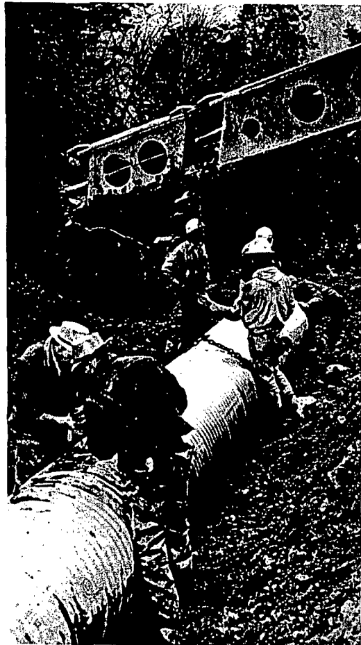
Boom of backhoe is used as crane for lifting sections of culvert into place while repairing washout near Richardson Grove.
