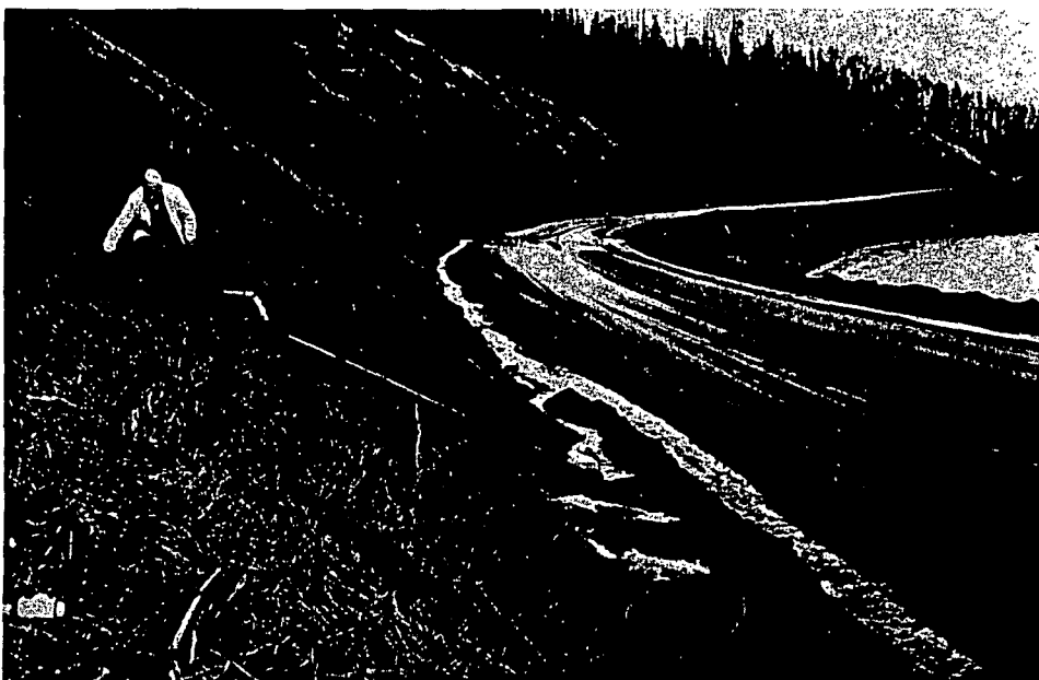
ABOVE: This paving damage was caused by pressure of sliding material on slope at right, forcing its way between road surface and foundation. BELOW: Man in photo has right hand at high-water mark which South Fork of Eel reached here near Phillipsville. This stretch of freeway, recently completed, was constructed five feet above high-water line of 1955 flood.
