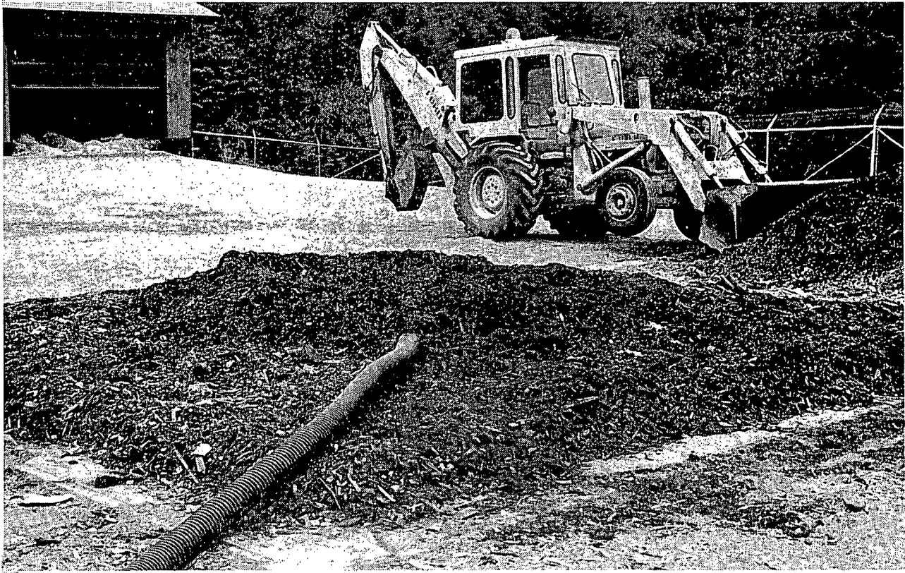
Figure 7: The perforated pipe is covered with coarse wood chips to help prevent the liquid waste/bulking mixture from clogging the holes in the pipe and reducing air flow through the pile.
