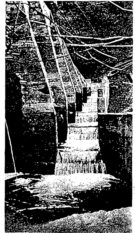
FIG. 41. A fishway at Benbow Dam. There are alternating miniature falls and resting pools. Photograph by John Spencer.
