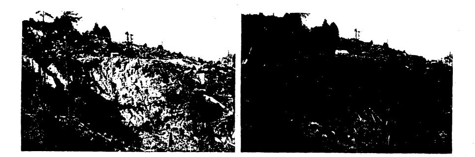
PHOTOS 2 and 3. (September and December, 1978): Log landing in the Miller Creek drainage on the C-line before and after rehabilitation by heavy equipment and manual labor crews. The outer part of the landing failed about 5 years ago and left a perched scarp of soil and organic debris above the stream. Heavy equipment removed the perched material, recontoured the slope, and manual labor crews then planted and wattled the slope (see text).
