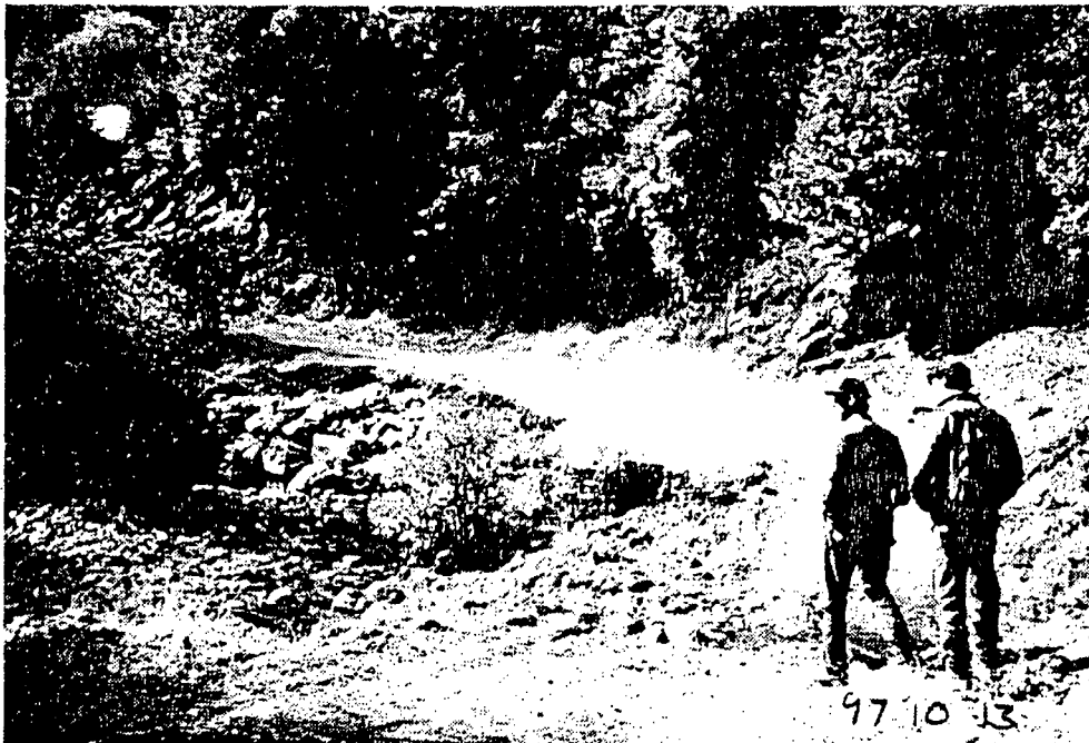
Left: Curtis Ihle of NEAP and Project worker Jesse Russell inspect the "rocked ford" at Simmonds Gulch on Maple Basin Road, a salmonid stream crossing suffering from continual stream bank erosion and lack of vegetation. Salmonid fingerlings were seen in this puddle in the road in spring 1997.
