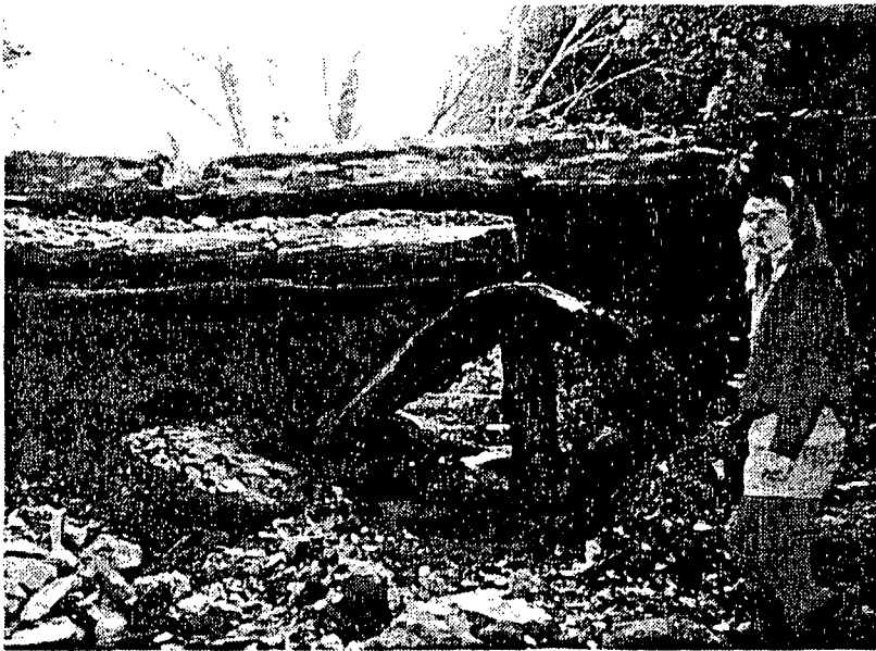
In summer 1997, Sky Ranch had to re-install the old culvert to keep the fire road open, while the Project sought funding and permits for a flatcar bridge.
