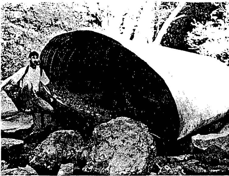
Left: The Sky Ranch Estates culvert on the main stem of Greenwood Creek, discovered by Jesse Russell (in the photo) and Dave Gurney during the 1996 Road Survey. The culvert had blown out several years in a row, sending tons of sediment into the Creek. The Sky Ranch Estates Association was required to keep the road open for fire and rescue access and couldn't afford the more permanent solution of a bridge. When NEAP funds became available to the Project in fall 1997, a solution was formulated.
