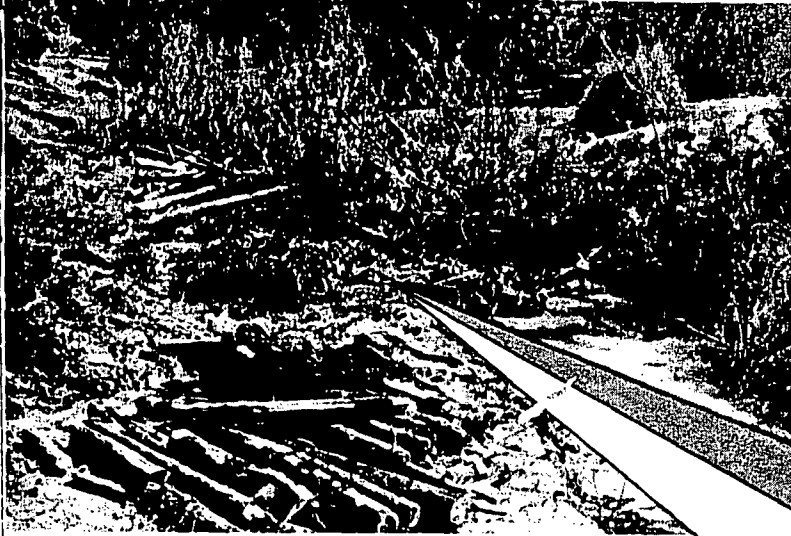
The contrast. A cleared area in the foreground points up the difference in the solidly jammed section of Olds Creek just upstream. DFG photos with this article by Gerald Holman.
