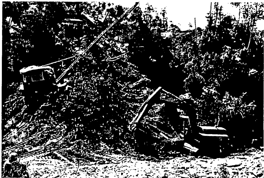
Fig. 57. Hydraulic excavator, dragline crane and crawler tractor excavating and disposing of material stored behind the log jam, Copper Creek.
