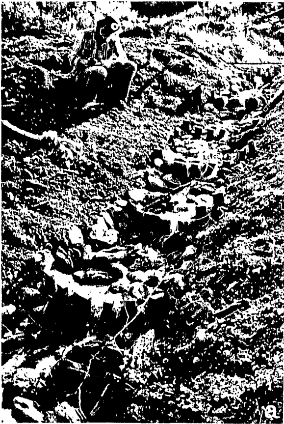
Fig. 9 (above). Hand-placed and secured rock armor in two small channels (A and B) excavated through the former L-1-5 logging road.
