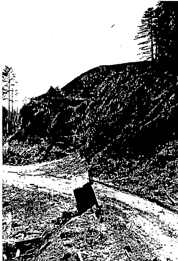
Fig. 23. Alluvial fan created by runoff from improperly drained yarder pad above the M-7-5-1 road.
