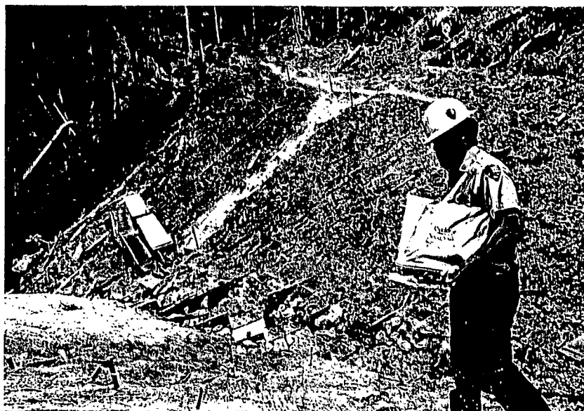
Fig. 41. Alder and grass seed being hand spread at stream crossing R7.
