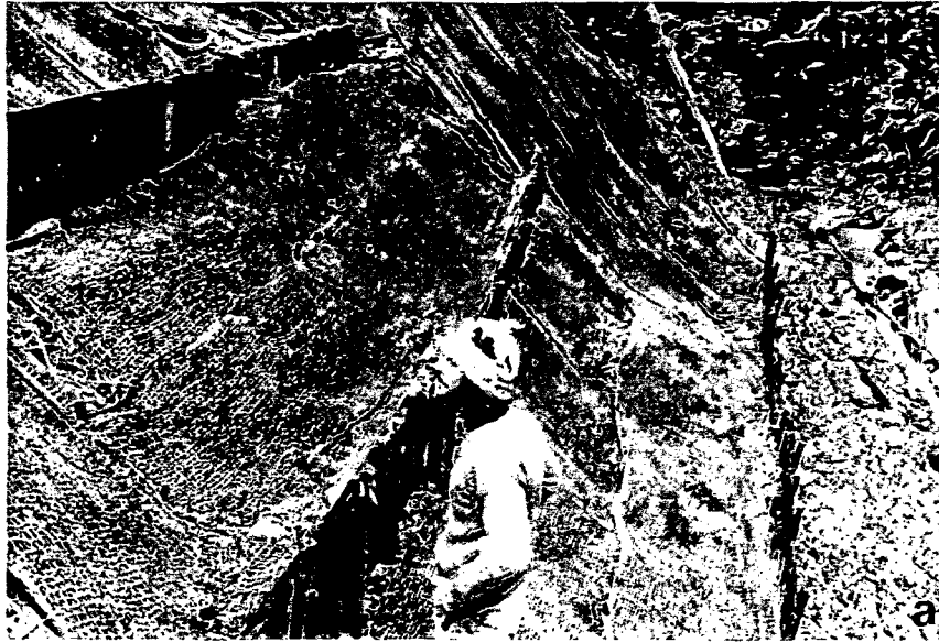
Fig. 38. Ravel catchers and jute-covered straw mulch on crossing R9. A) ravel catchers and jute-covered straw mulch were placed on the steep right bank of excavated stream crossing R9. B) following a small cutback failure on the former logging road at the top of the excavation, soil and rock passed over the jute (with no apparent damage) and either filled or toppled the ravel catchers.
