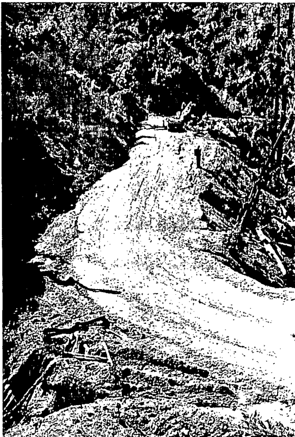
Fig. 3. Tension cracks in the fill slope, L-1-5 logging road.
