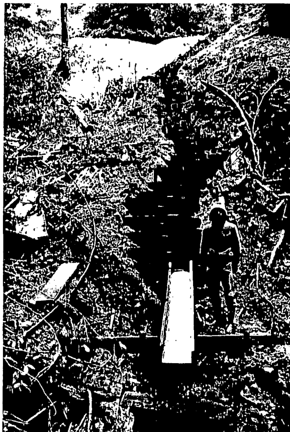
Fig. 35. Protection of a steep, rilled slope near crossing R9 using small checkdams and a flume with energy dissipater. In retrospect, this treatment was judged excessive for the comparatively small amount of runoff and erosion which would have occurred. As with this case, runoff volumes from treated areas and former springs are often difficult to predict.
