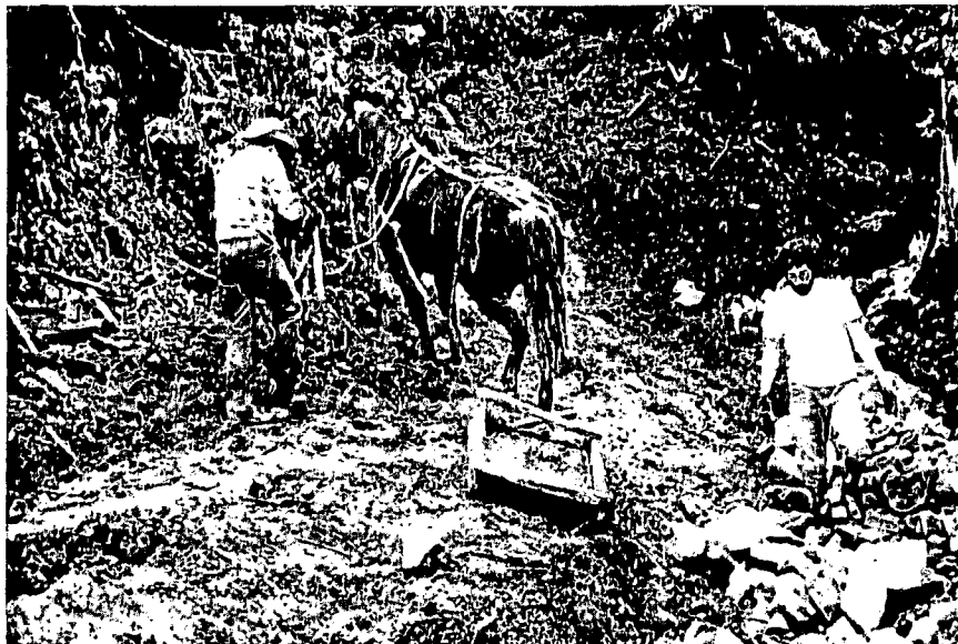
Fig. 76. Horses and sleds moving rock for stream crossing armoring in the middle Copper Creek contract area. The rocks were then placed in the channel by hand. In the smaller streams, hand-placed rock armor was generally successful in controlling post-rehabilitation erosion.
