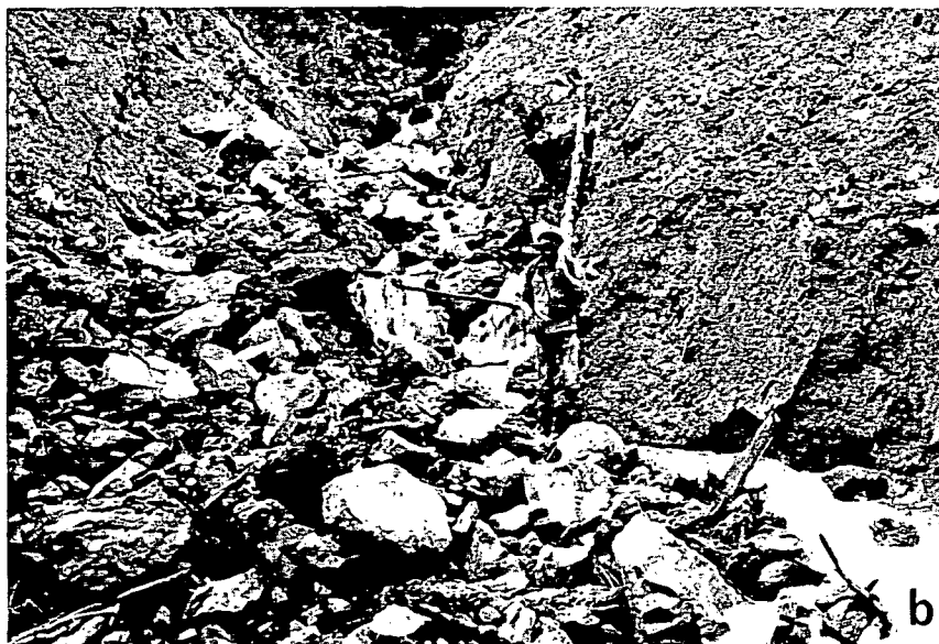
Fig. 31. Erosion of rock armored stream crossing R6. Sediment loss was caused by the presence of oversized rocks which diverted flow into and caused undercutting of the adjacent channel banks. Crossing R6 A) before heavy stream flows (October 1979) and B) after several winters (July 1982).
