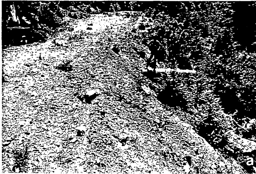
Fig. 65. Successful, major stream crossing excavation. A) intact crossing prior to rehabilitation work, note workers standing on the culvert inlet and outlet, and largely unvegetated road surface; B) same view of crossing taken immediately following excavation work; note the basal flair on the exposed redwood stump which indicates the original ground surface (stream channel bottom) was successfully exhumed; C) same crossing after three and one-half years; because the channel was excavated down to the original ground surface, there has been little erosion of the streambed following rehabilitation.
