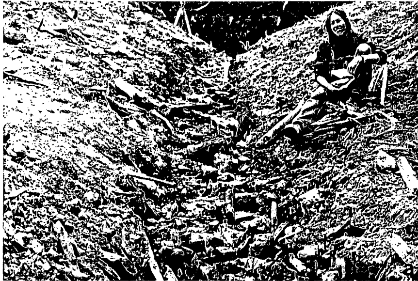
Fig. 17. Serial photographs of channel changes at the excavated stream crossing R1. Even though the crossing had not been fully excavated, abundant concentrations of organic debris buried in the fill helped minimize subsequent channel erosion. Figure 17A: October 1979; Figure 17B: June 1980.
