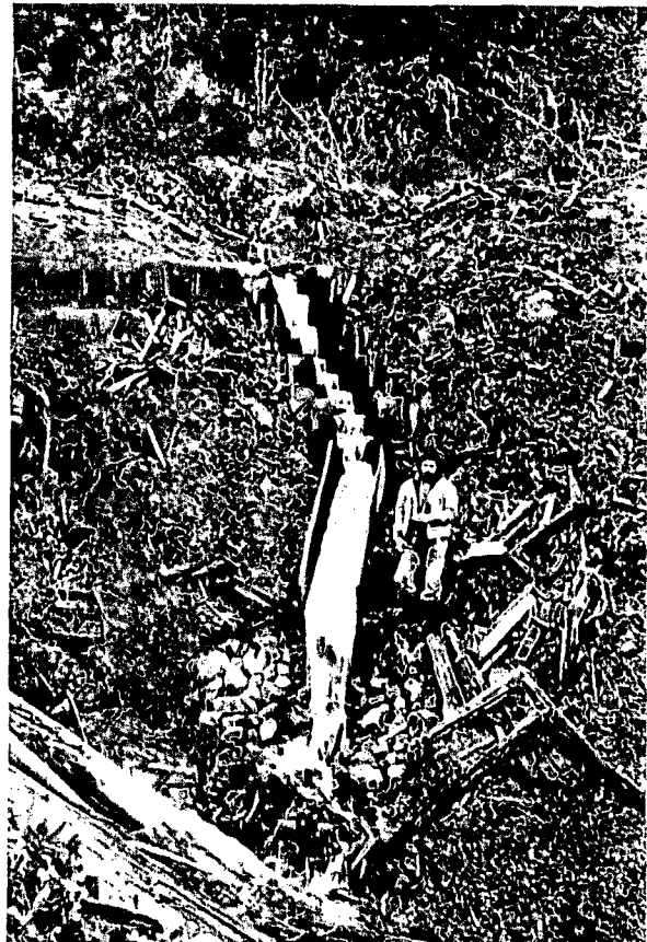
Fig. 9 (above). Hand-placed and secured rock armor in two small channels (A and B) excavated through the former L-1-5 logging road.
