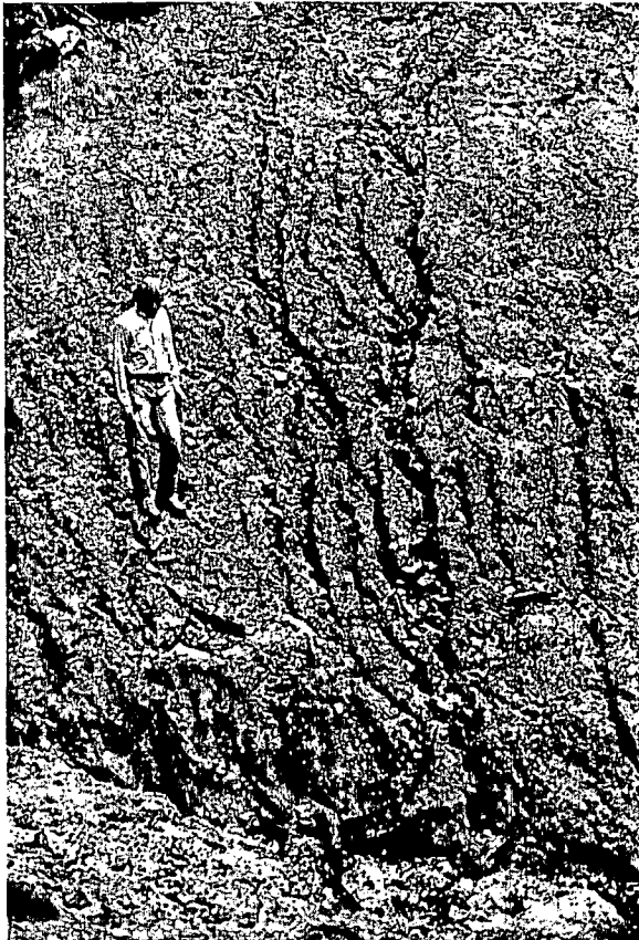
Fig. 34. Early winter rilling on the steep side slope of excavated stream crossing R7. Photo was taken prior to application of straw mulch and jute netting (October 1979).
