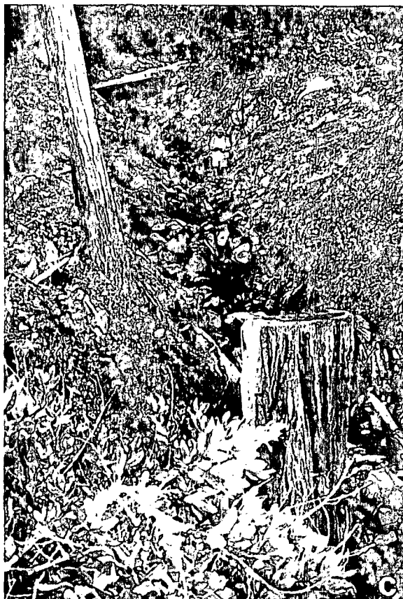
Fig. 66. Excavation of logging road stream crossings using a hydraulic excavator. A) initial excavation of the outboard edge of the crossing is done while the excavator sits on the road surface; B) as the former bed and banks of the stream channel are exhumed or reconstructed, the excavator moves to one side and passes material onto the road surface directly behind it; C) same crossing after approximately four years, note minor channel adjustment and the lag deposit of coarse rock armor which has developed in the streambed.
