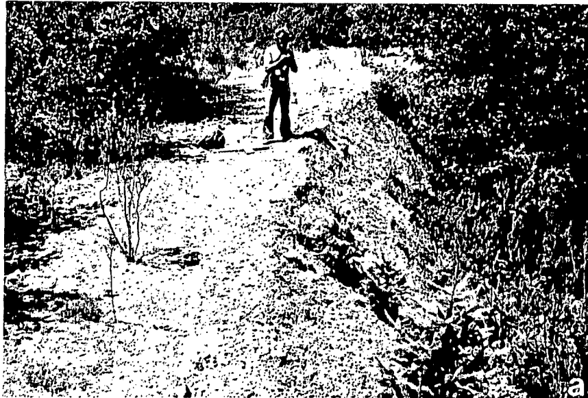
Fig. 61. Rehabilitation of a secondary logging road. A) after ten years of abandonment, but prior to rehabilitation treatments — note lack of re-vegetation on the road surface; B) immediately following road ripping and construction of cross road drains. Decom-packed road has also been lightly mulched with straw.
