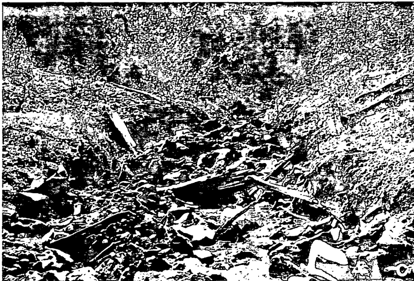
Fig. 79. Changes at an excavated stream crossing following rehabilitation. A) view upstream during the first winter flows; B) same view after first winter; note minor channel downcutting, considerable widening and the removal of under-sized rocks used in the channel armor; C) after the second year, the channel has downcut an additional foot and widened several more feet in response to sustained high flows during the winter (note the organic debris being exhumed); D) in 1983, 4 years after treatment, large boulders are now being exhumed as the stream finds its original, stable bed. Note also that widening continues to occur and young trees topple into the streambed.
