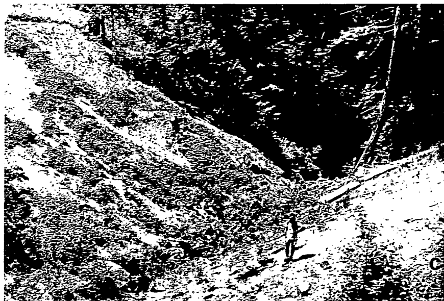
Fig. 43. View of the excavation and revegetation of stream crossing R7, M-7-5-1 logging road. A) M-7-5-1 logging road before rehabilitation and excavation of the stream crossing material (note drop inlet to culvert), May 1979; B) after channel excavation; note straw and jute netting on the left bank, sediment troughs on right bank, and checkdams in channel (January 1980); C) one year, eight months after rehabilitation, showing patchy alder growth from seeding (left bank) and growth of planted alder seedlings and grass (right bank) (May 1981); D) two years, nine months after rehabilitation, showing dramatic alder growth and essentially equal success (in both height and number) of seeded and planted alder at this locality (July 1982); E) three years, ten months after rehabilitation, showing complete closure of new canopy over excavated stream crossing (August 1983).
