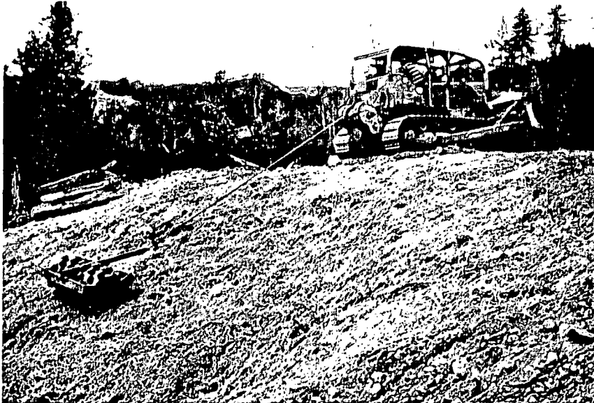
Fig. 63. Spiked roller used to punch straw into loose soil on steep, newly exposed slopes. An alternate treatment used on steep, inaccessible slopes elsewhere was the application of jute netting over the straw mulch (for example, see Bridge Creek Unit 79-2).
