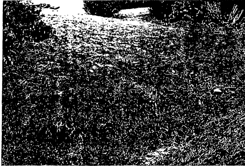
Fig. 80. Straw mulch, applied at 6000 pounds per acre, was found to be the most cost-effective treatment to control surface erosion from bare soil areas on 1979 rehabilitation units.
