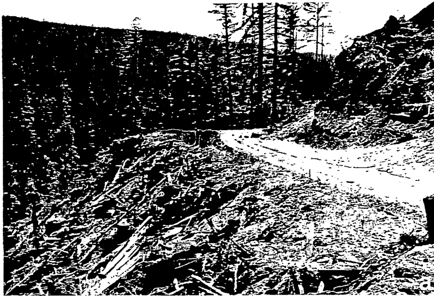
Fig. 30. Serial photographs depicting the treatment and recovery of landing 2. Outsloping and debris removal along several portions of the M-7-5-1 road was expensive but resulted in reduced erosion and rapid revegetation. A) landing 2 before heavy equipment rehabilitation treatment (June 1979); B) after debris removal, outsloping and the natural invasion of alder seedlings approximately 3 years later (July 1982); C) roughly 4 years after treatment (August 1983).
