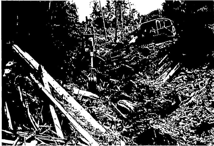
Fig. 5. Tractor and backhoe excavating skid trail stream crossing.
