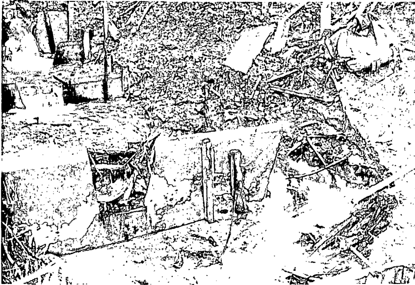
Fig. 12. Washed out checkdam. Organic debris plugged the spillway, diverted streamflow against the left bank and caused lateral scour around the structure.
