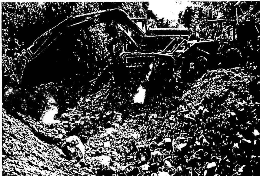
Fig. 62. Rock armor being placed in excavated stream crossing by excavator and loader. Rock used to protect newly excavated stream channels was derived locally for some crossings and from the Copper Creek rock pit for others (see Figure 54).
