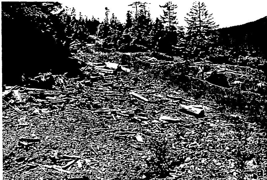
Fig. 71. Natural revegetation of a decompressed road surface. A) before rehabilitation, the former road surface showed little natural revegetation in the 10 years following its abandonment; B) same area immediately following decompression and outslowing (November 1979); C) four years later (September 1983) the site has been covered with naturally invading coyote brush. Revegetation of this hot, dry southwest facing slope contrasts sharply with the cool moist areas in Bridge Creek (unit 79-2) which were invaded by rapidly growing alder.
