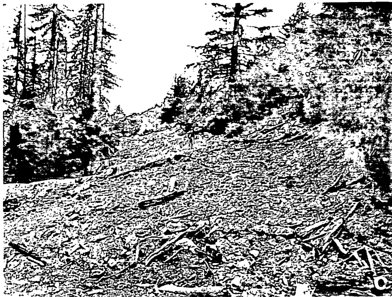
Fig. 6. Outsloping a segment of the L-1-5 road. A) diagrammatic sketch of road outsloping showing excavation of road fill and burial of inboard ditch and cutbank, B) before heavy equipment treatment (May 1979), C) immediately after outsloping and D) two year later (June 1983). All photos taken from the same viewpoint.
