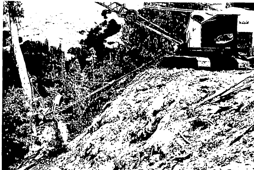
Fig. 55. Dragline crane excavating soil and organic debris from the outside edge of a log landing.
